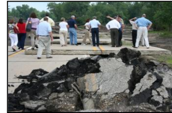
Members of the Rebuild Iowa Advisory Commission survey a roadway heavily damaged by floodwaters near Oakville.
