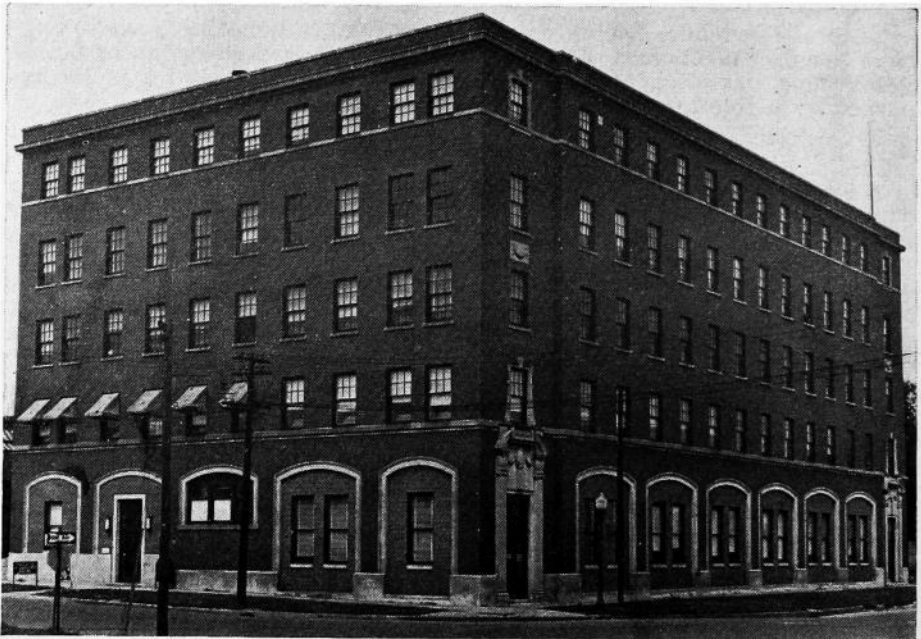
OFFICE AND LAB BUILDING AT EAST SEVENTH AND COURT Bought and remodeled at a cost of $541,972.
