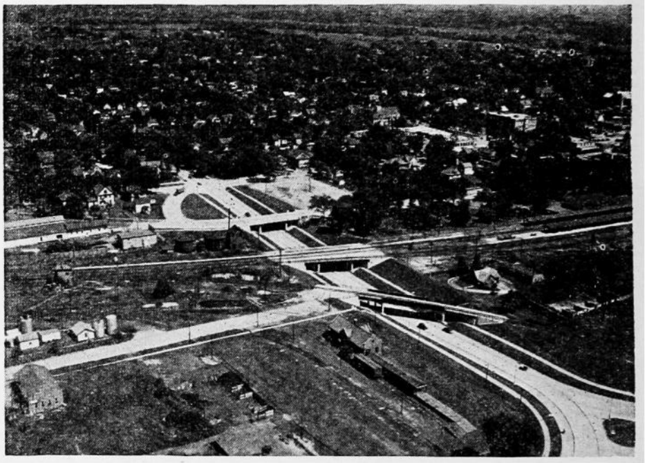
Subway and Traffic Separation Project at Ames
