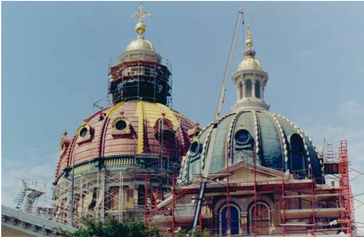
1999 gilding in progress. (Photo: RDG Planning & Design)
