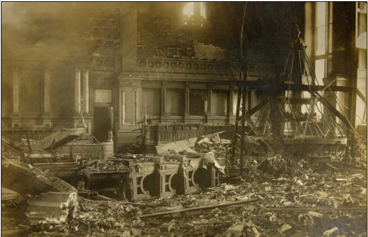
The picture above shows the Iowa House of Representatives Chamber in 1904 before the fire. Below is a picture of the Iowa House of Representatives Chamber's damage after the fire. The flames burned through the ceiling and caused much of it to collapse to the floor below, while the lower areas of the building were damaged by smoke and water.
