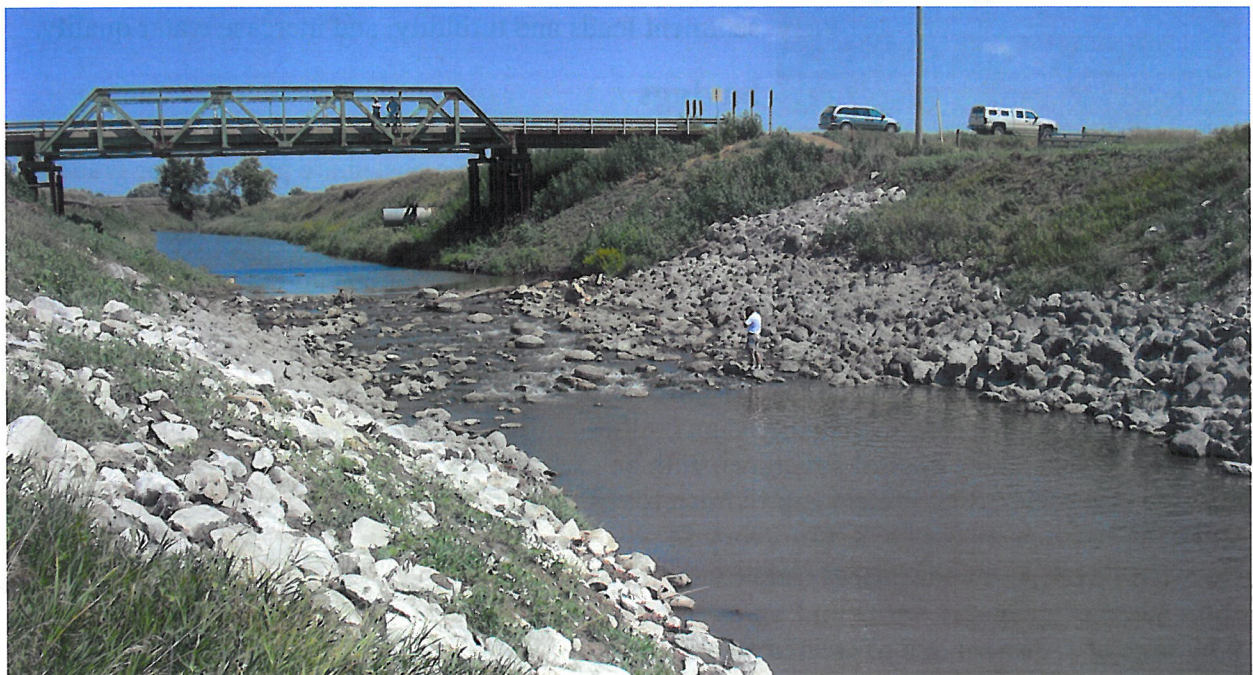
Sheet pile weir with a 20:1 grouted riprap slope, designed to allow fish passage, in Montgomery County.
