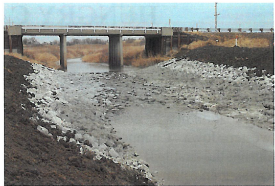
Sheet pile weir with a 20:1 grouted riprap slope in Crawford County.
