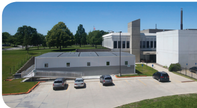
Current VDL Facility Entrance
