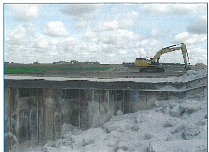
Construction underway at a CREP wetland located in the Boone River watershed
