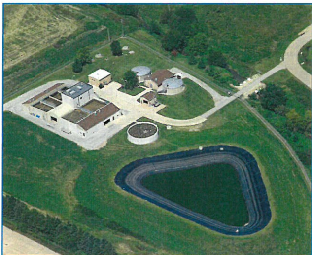
City of Eldridge wastewater treatment plant. Photo Courtesy of Mayland Aerial Photography
