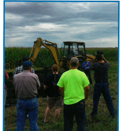
Saturated buffer installation in Dallas County as part of RCPP project
