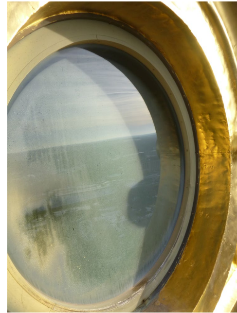
Photo 64 Condensation on circular window interior.
