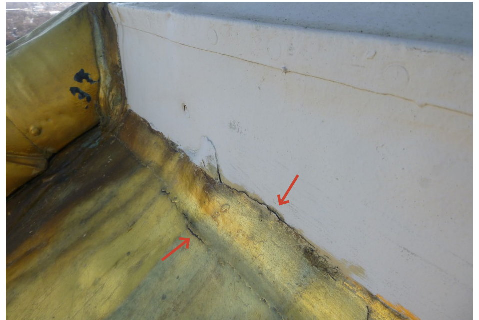
Photo 53 Lead fillet at transition between dome roofing and lantern skirt cladding; note separation between fillet and roofing/cladding.
