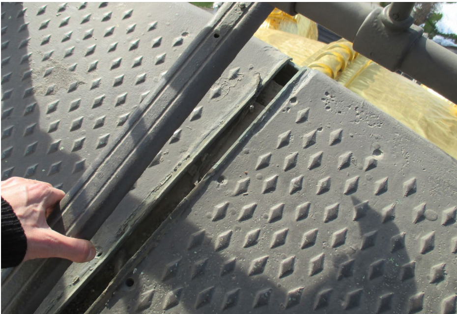
Photo 36 Unsecured cover; corroded framing is visible below.
