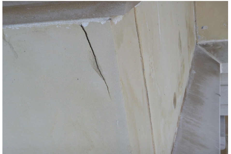
Photo 74 Typical isolated masonry crack.
