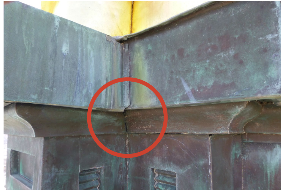
Photo 66 Typical open seams in non-skyward-facing joints of copper entablature at base of dome.
