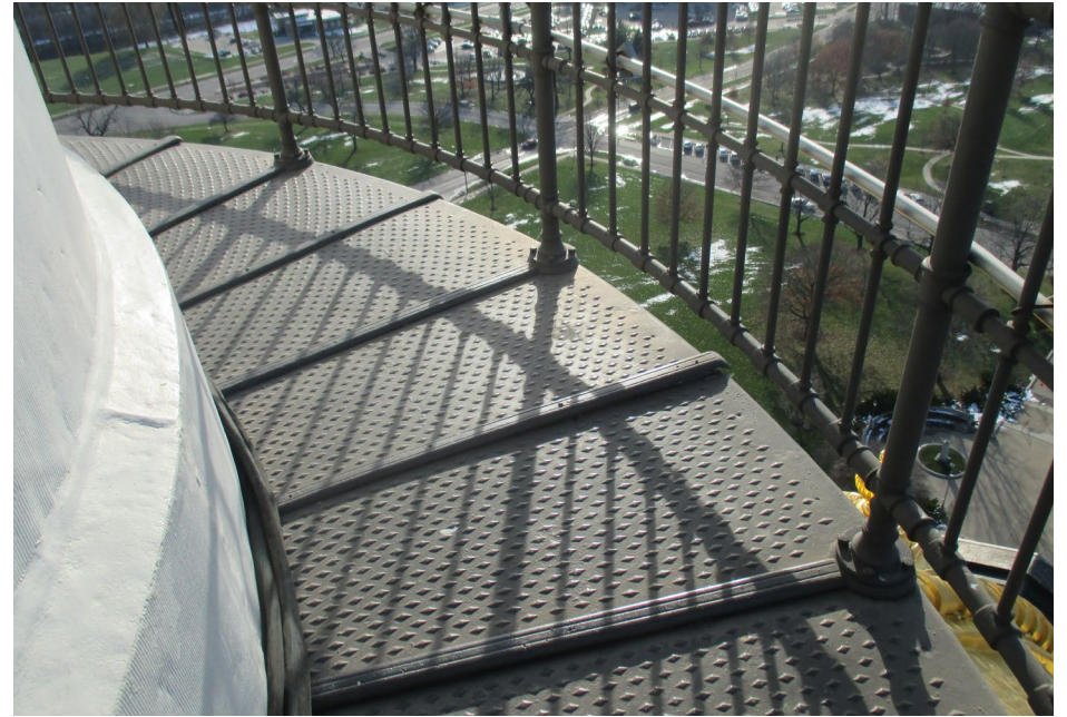
Photo 35 Observation deck planks, covers, and guardrail.
