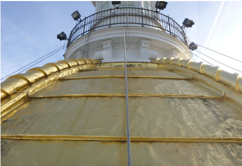
Photo 48 Typical gilded dome roofing.
