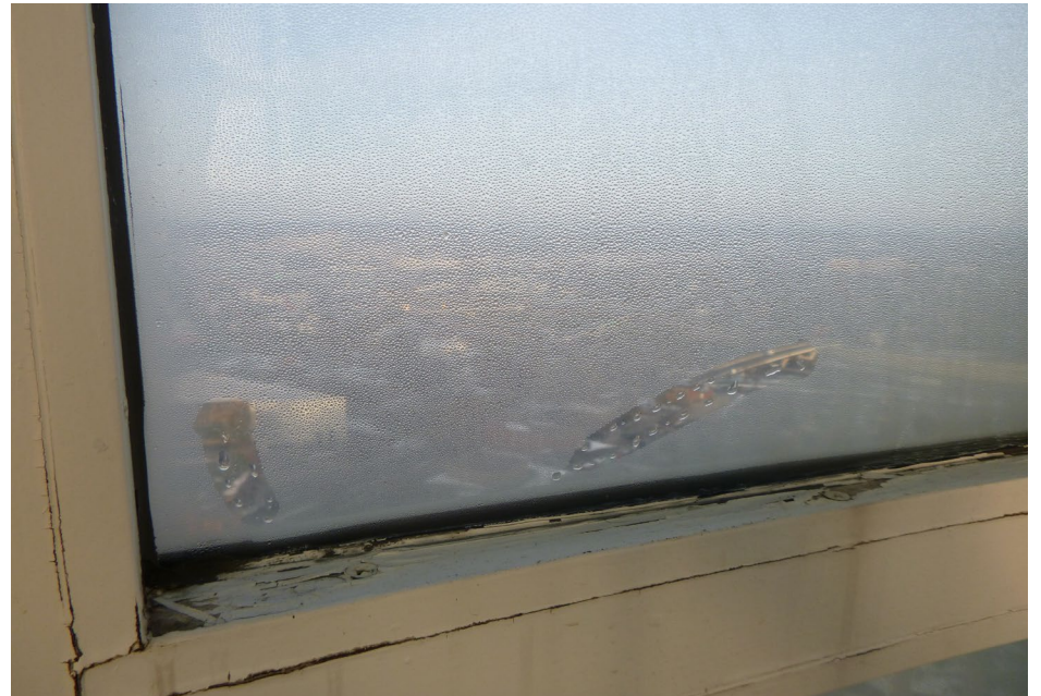
Photo 9 Lantern window condensation.
