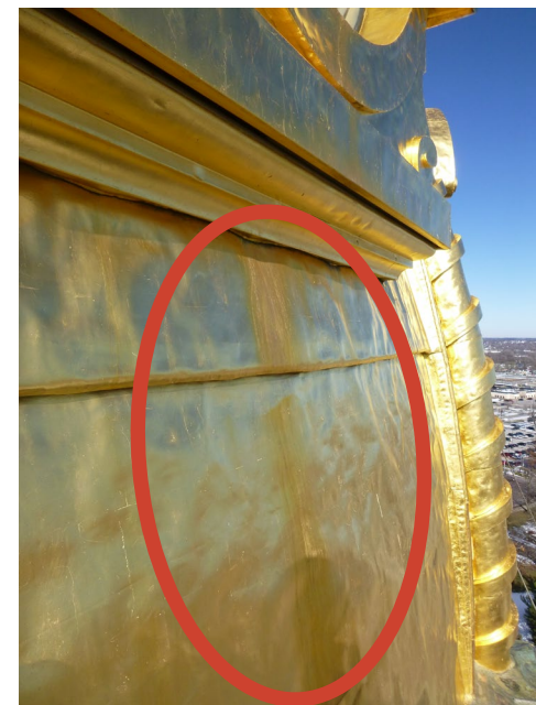
Photo 62 Water stains originating from base of eyebrow dormer.
