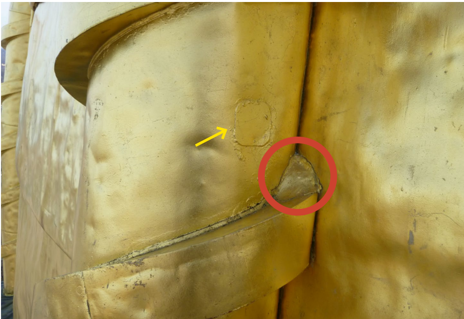
Photo 52 Repair patch (yellow) and lead cant (red).
