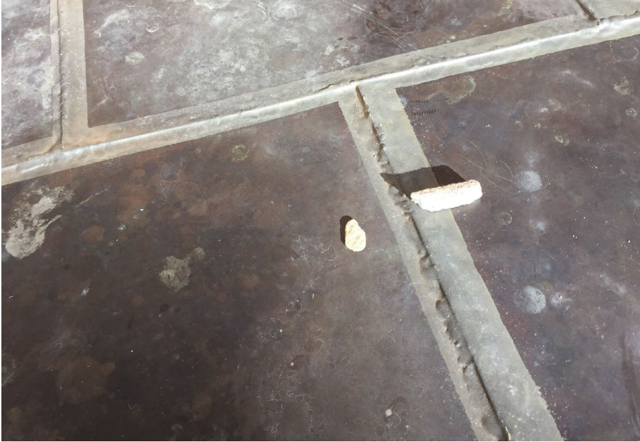
Photo 87 Stylobate level - Masonry joint fallen from above on copper flatlock.
