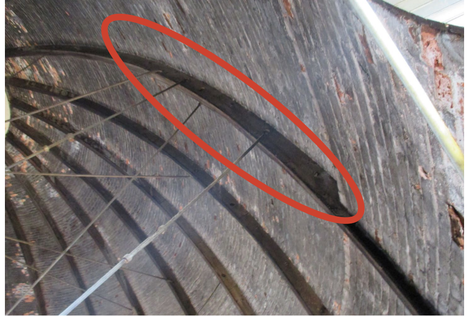
Photo 23 Brick shell and ribs; note wood blocking through-bolted to rib webs at upper single-wythe shell area.
