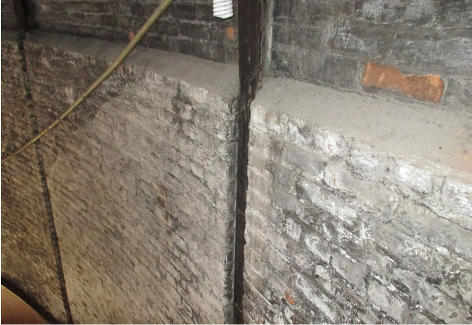
Photo 22 Brick shell's step from two to three wythes.
