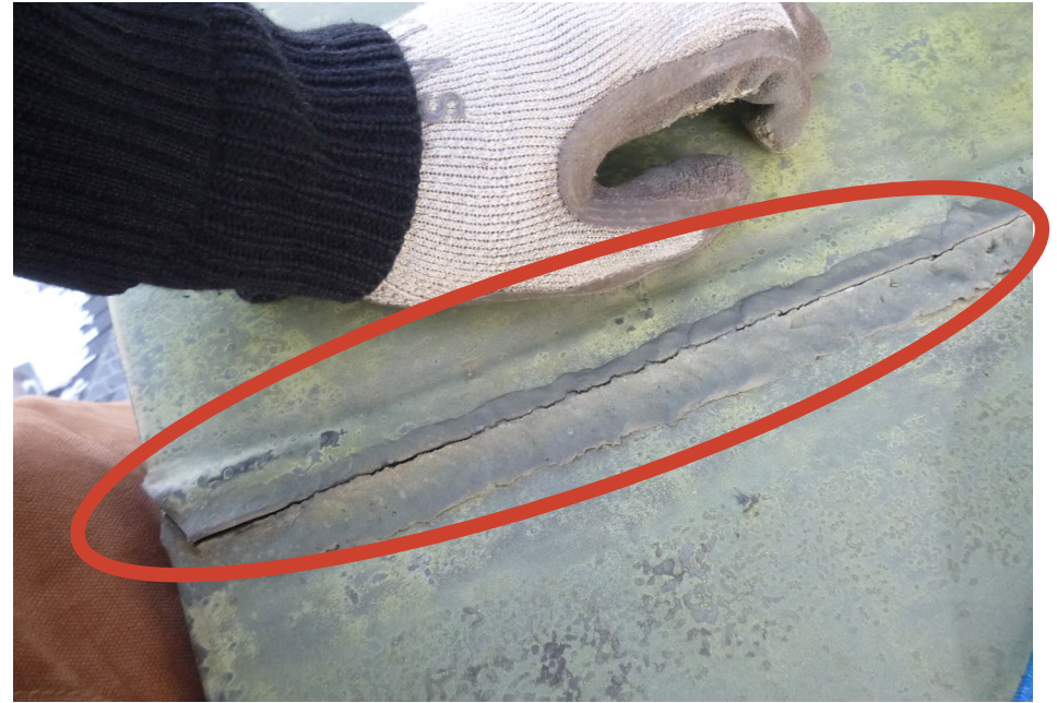
Photo 68 Cracked solder joint in upper cornice flashing.
