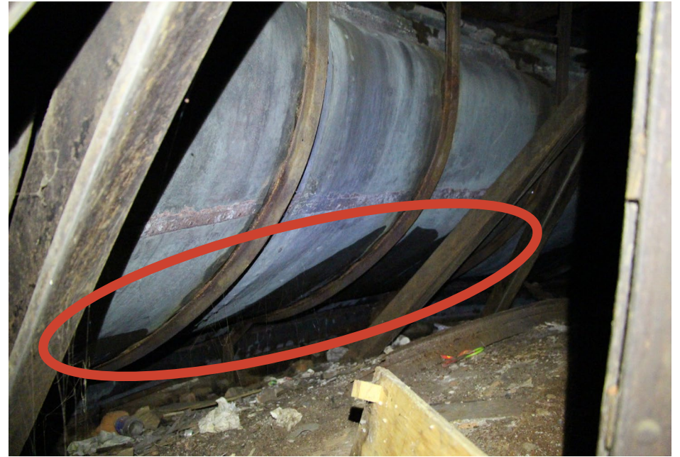
Photo 15 Condensation observed on the underside of the lantern sheet metal cladding.
