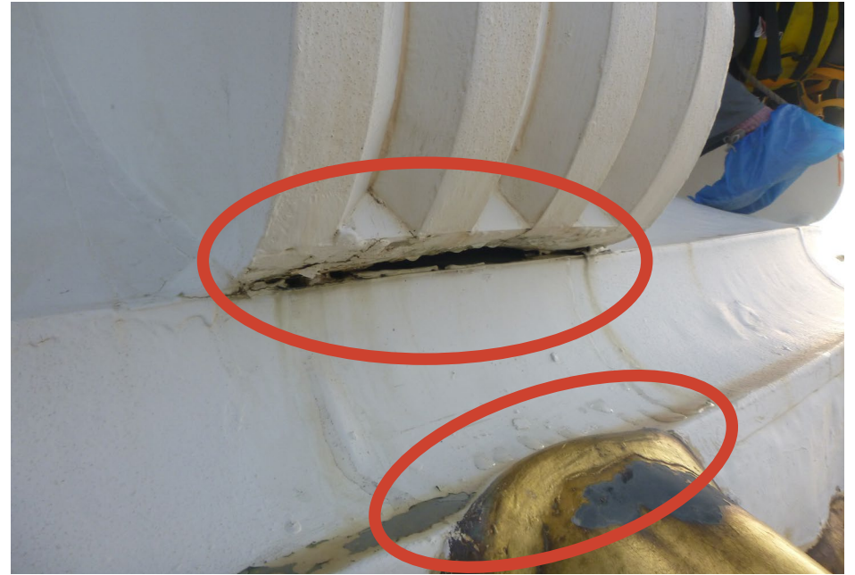
Photo 43 Typical gap at base of bracket; note water on cladding below (several days after any rain/snow).
