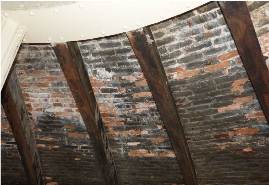
Photo 24 Typical brick deterioration at top of dome.
