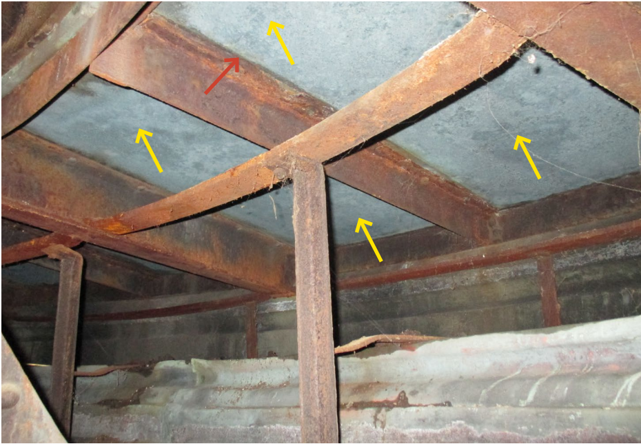
Photo 14 Framing below observation deck planks (yellow arrows) is corroded; note built-up rust scale at WT member directly below planks (red arrow).
