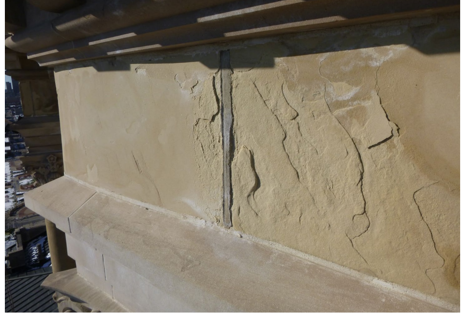
Photo 72 Delamination at sandstone frieze within lower cornice entablature.
