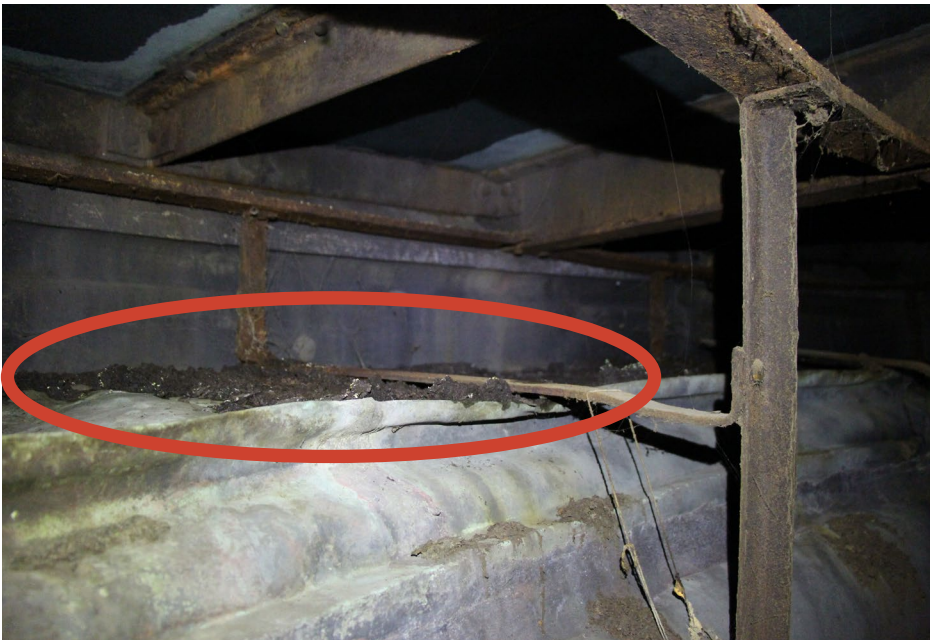
Photo 16 Wet and debris-filled soffit within the lantern attic.
