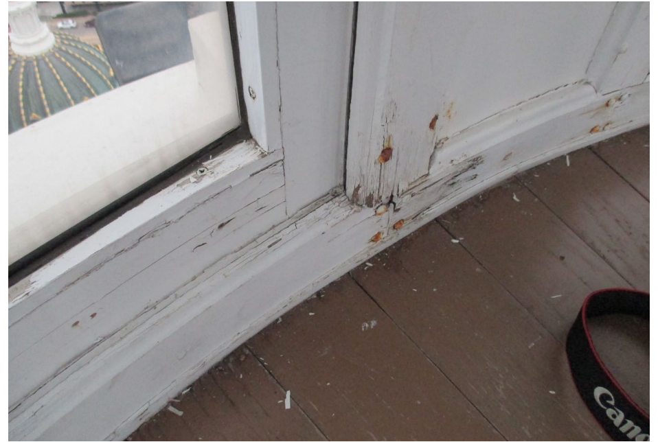
Photo 11 Typical failing paint, deteriorated wood & corroding fasteners at lantern window sill.
