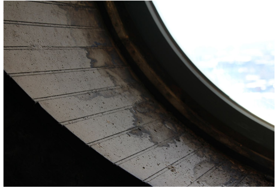
Photo 31 Water staining on wood finishes at interior of window.
