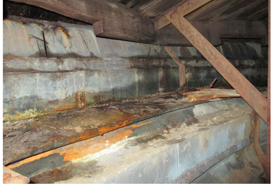
Photo 6 Condensation accumulation in the lantern dome soffit.
