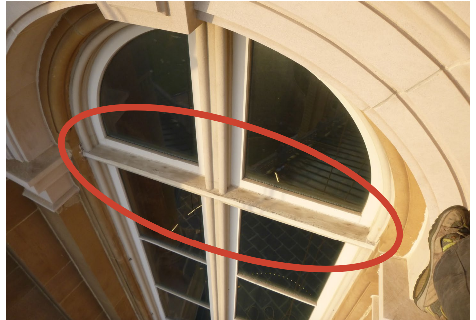
Photo 76 Typical drum window; note failing paint on horizontal wood framing members.
