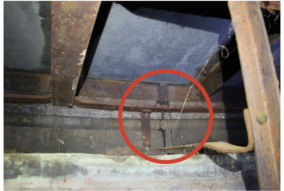
Photo 80 Prompt leakage produced at observation deck water test.
