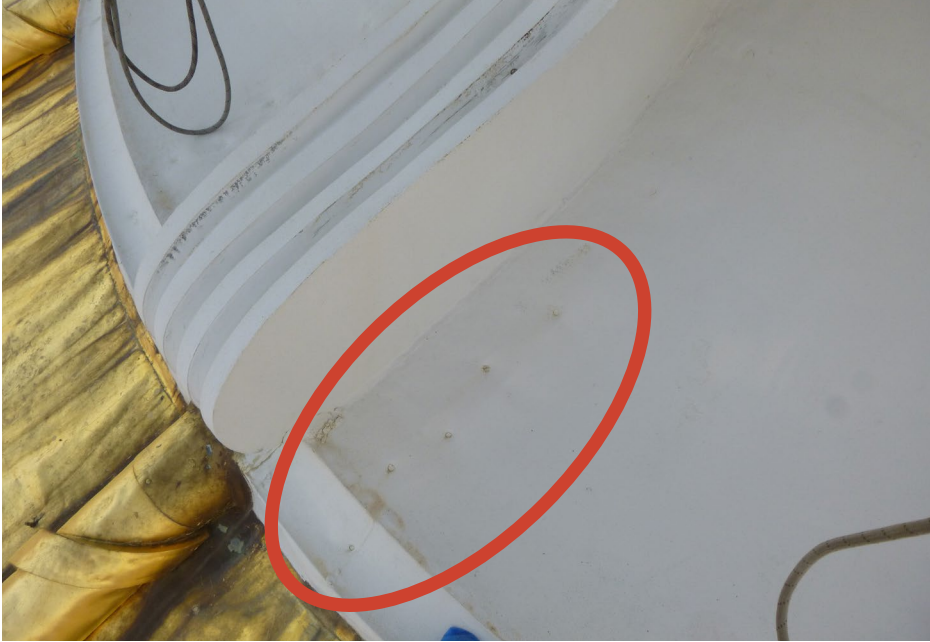
Photo 46 Fastener heads visible through coating.
