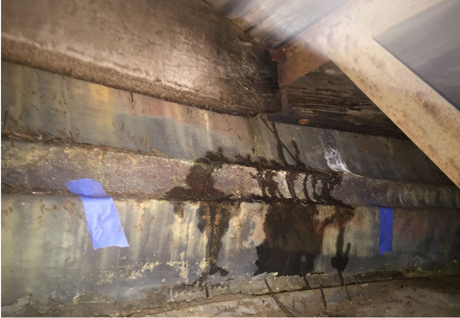
Photo 5 Leakage observed below lantern dome cornice during a rainstorm.
