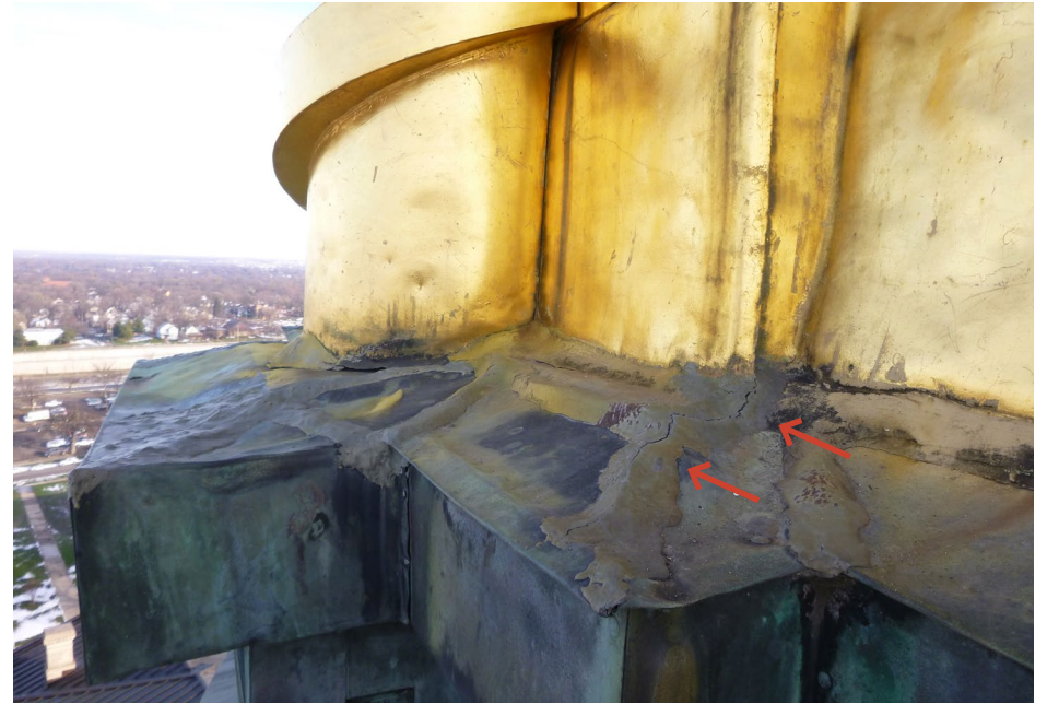
Photo 55 Small cornice at top of copper entablature at base of dome; note cracked solder joints.
