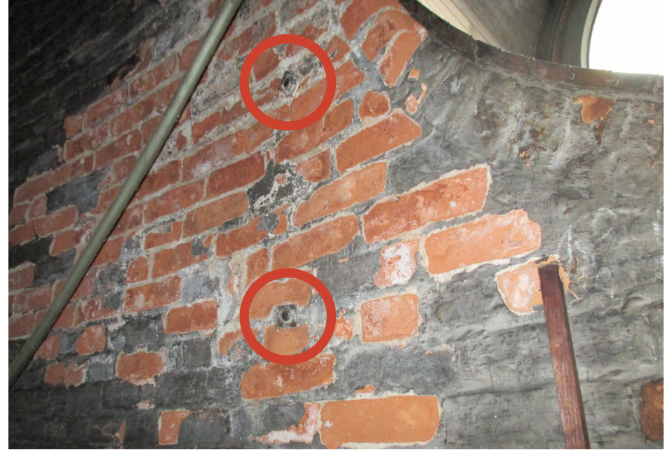
Photo 27 Closer view of brick deterioration shown in previous photo; note anchor heads from original construction.
