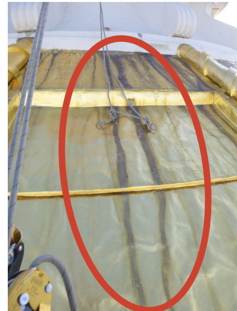
Photo 41 Stains on gilding below rust stain noted in previous photo.
