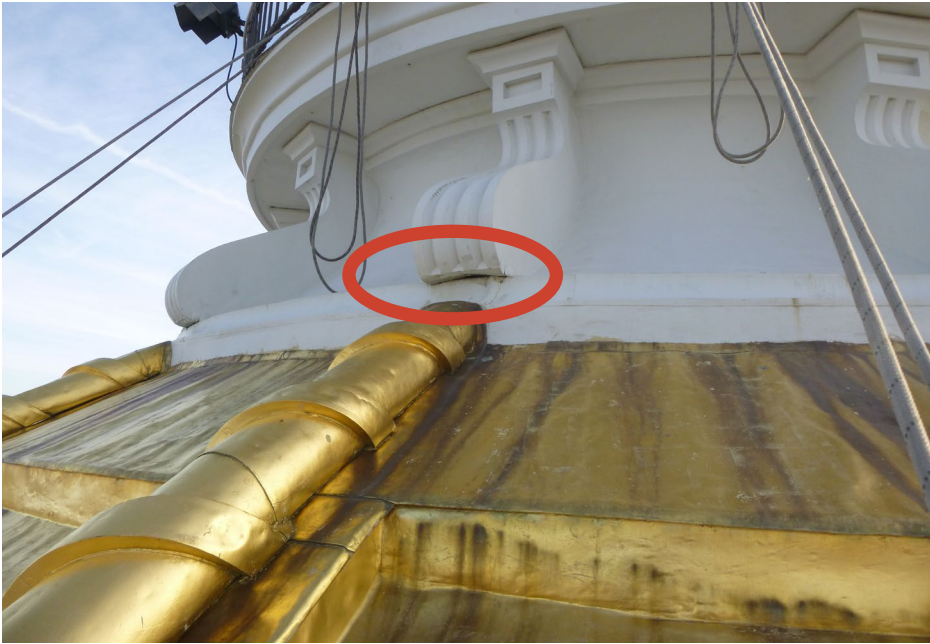
Photo 42 Lantern skirt and typical decorative sheet metal bracket.
