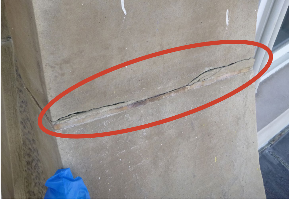
Photo 71 Failed mortar joints in brackets above lower cornice.
