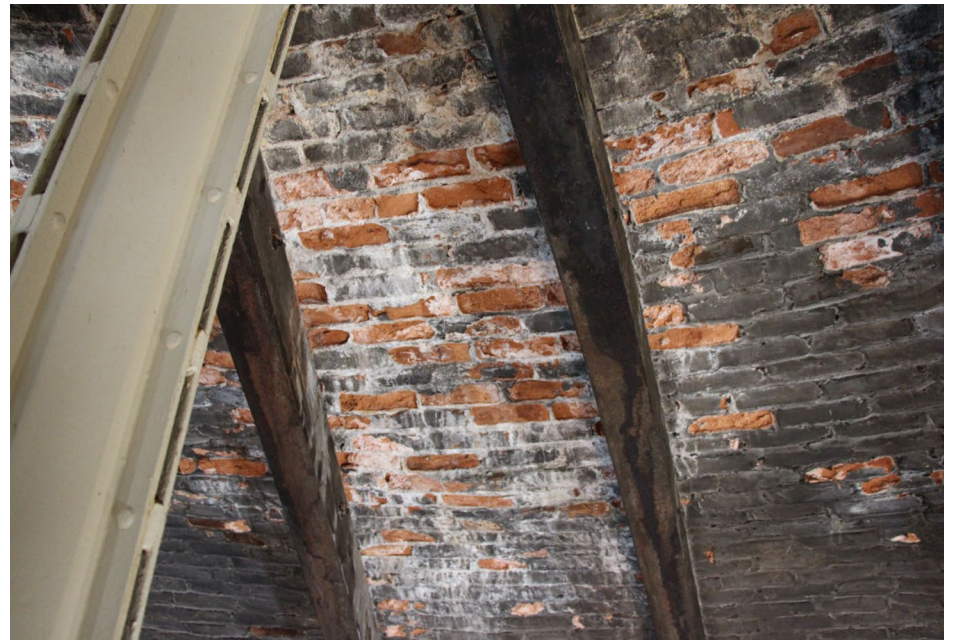
Photo 25 Brick deterioration and efflorescence at top of dome, southeast quadrant.
