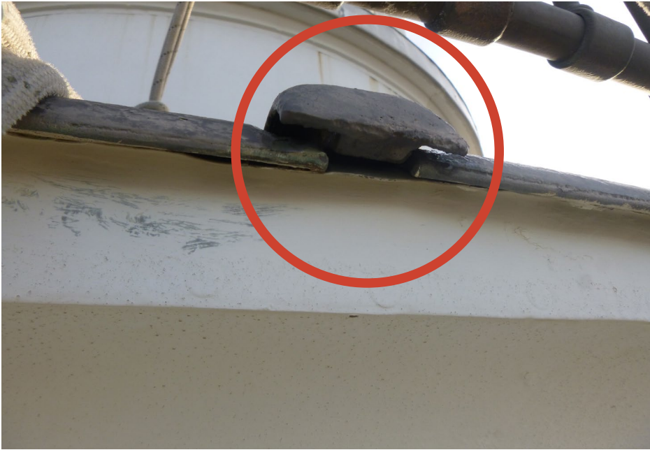
Photo 38 Edge of observation deck plank has limited overlap onto cladding below; note gap at end of cover.
