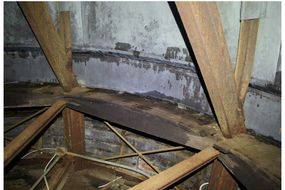
Photo 4 Condensation on backside of sheet metal cladding at the base of lantern dome.
