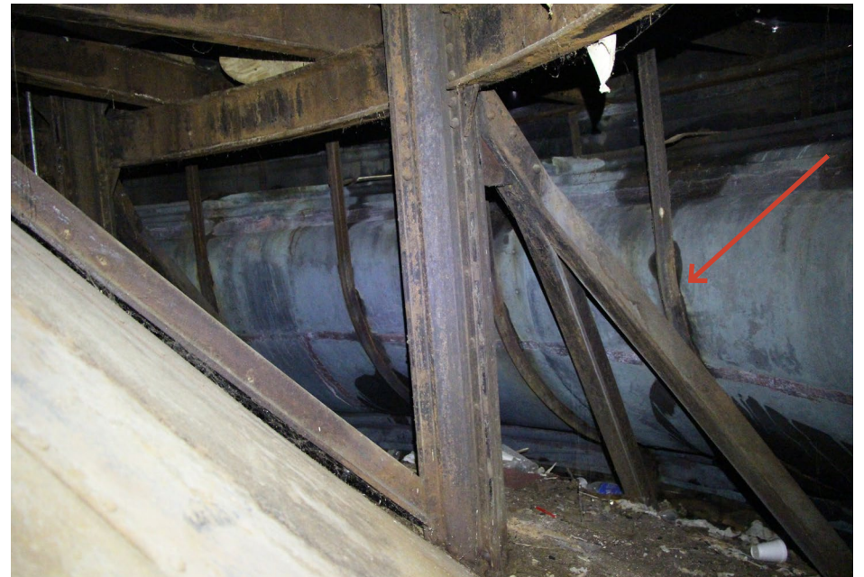
Photo 13 Metal framing & backside of sheet metal cladding (arrow) within the lantern attic.
