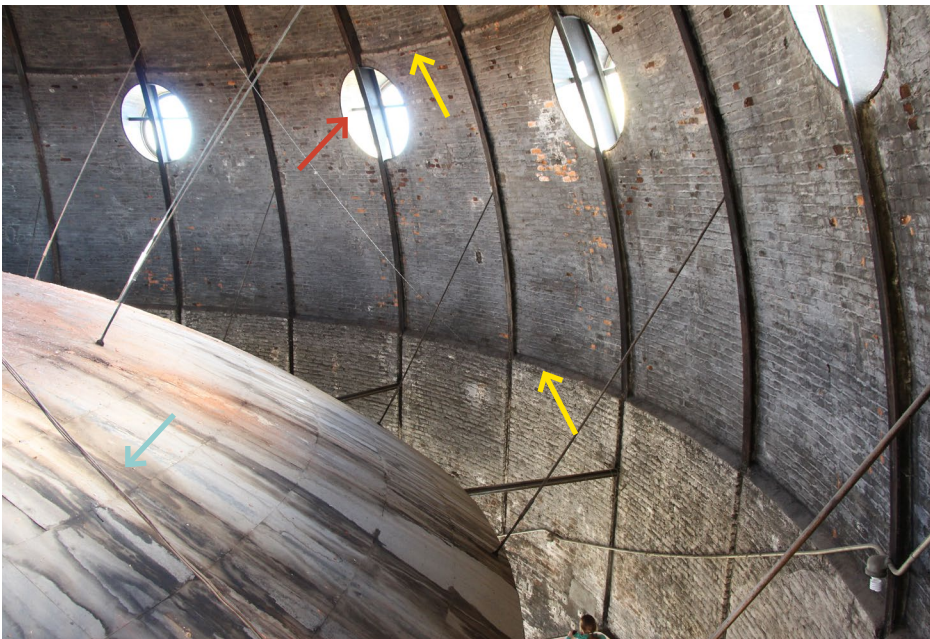
Photo 20 Typical brick shell and ribs; note steps in brick thickness (yellow), horizontal bracing visible at windows (red), and suspended sky dome with water stains and brick debris (blue).
