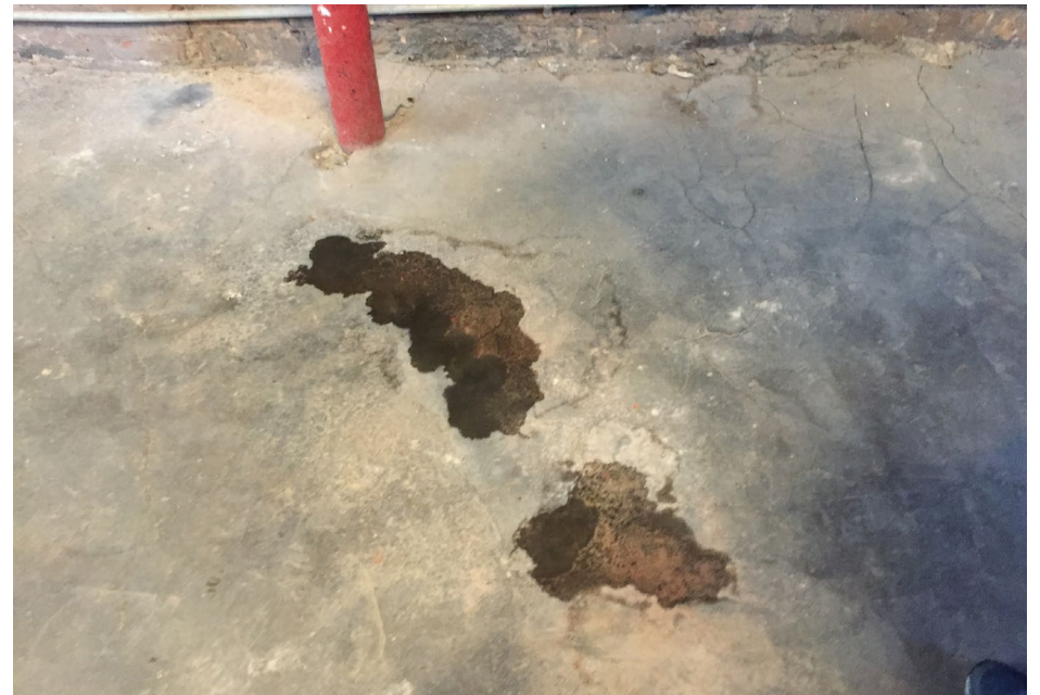
Photo 86 Stylobate level - Active water leak to the attic floor.
