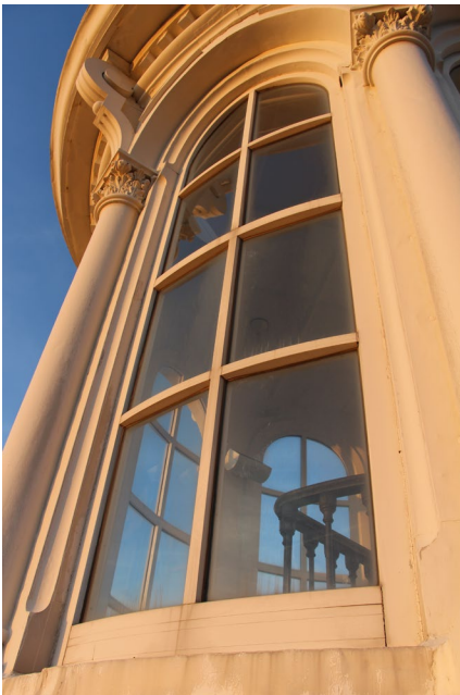
Photo 7 Typical lantern window.
