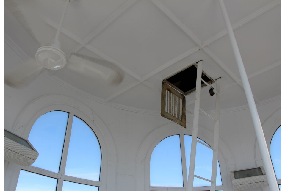
Photo 2 Lantern ceiling. Note grated hatch into lantern dome attic and ceiling fan.
