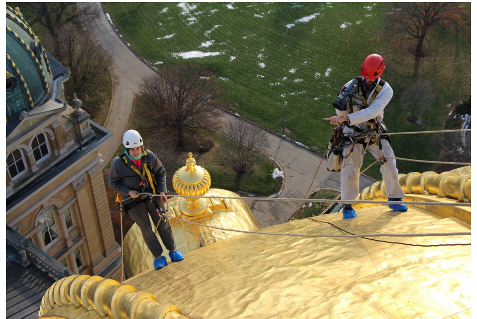
Photo 33 Industrial rope access used for exterior inspection.
