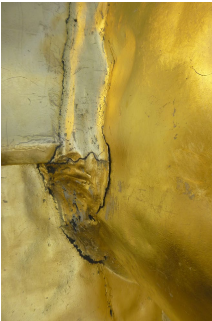
Photo 56 Splits and separation of typical lead fillet at eyebrow dormer.
