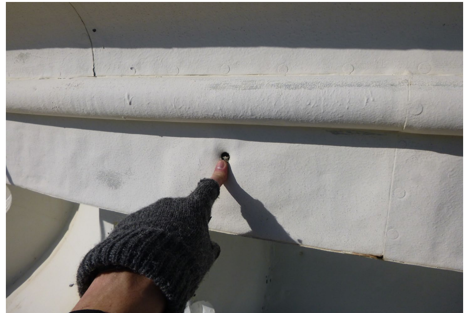
Photo 45 Hole in cladding directly below observation deck.
