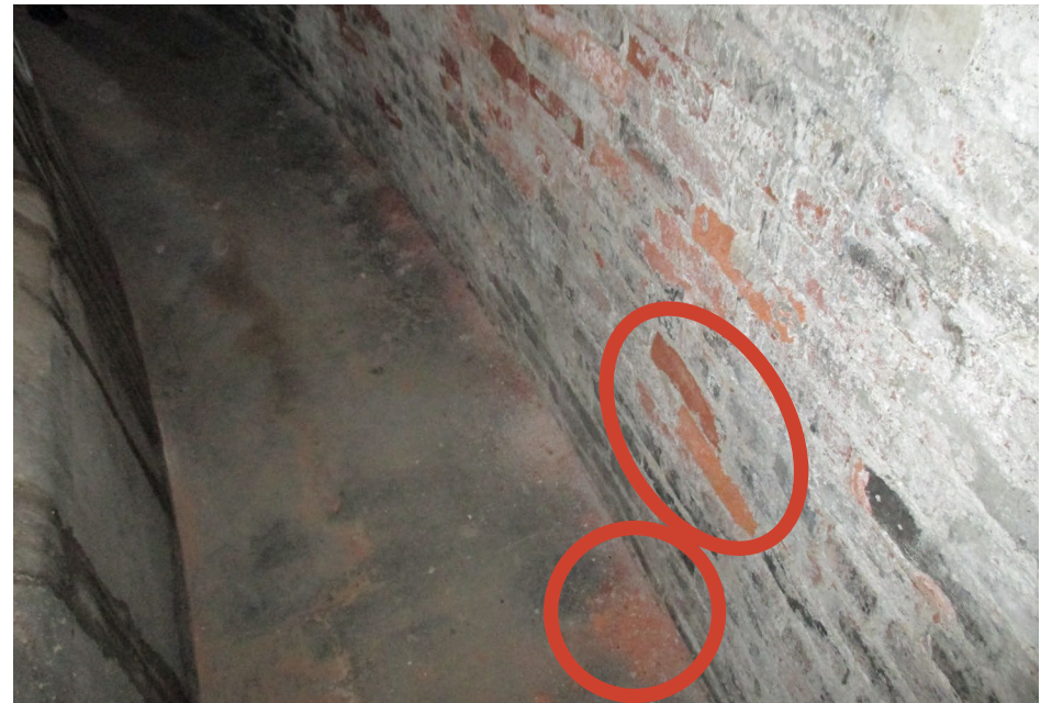
Photo 29 Isolated brick deterioration and debris at base of dome.
