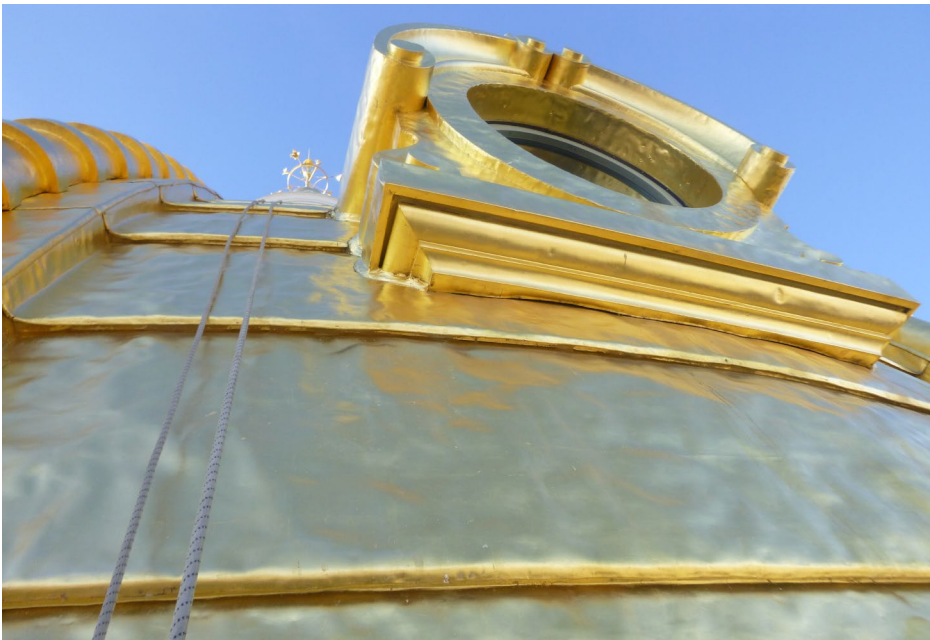
Photo 61 Typical dome eyebrow dormer viewed from below.
