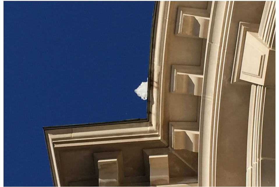
Photo 84 Ice about to fall from the base of Level J intermediate cornice copper.
