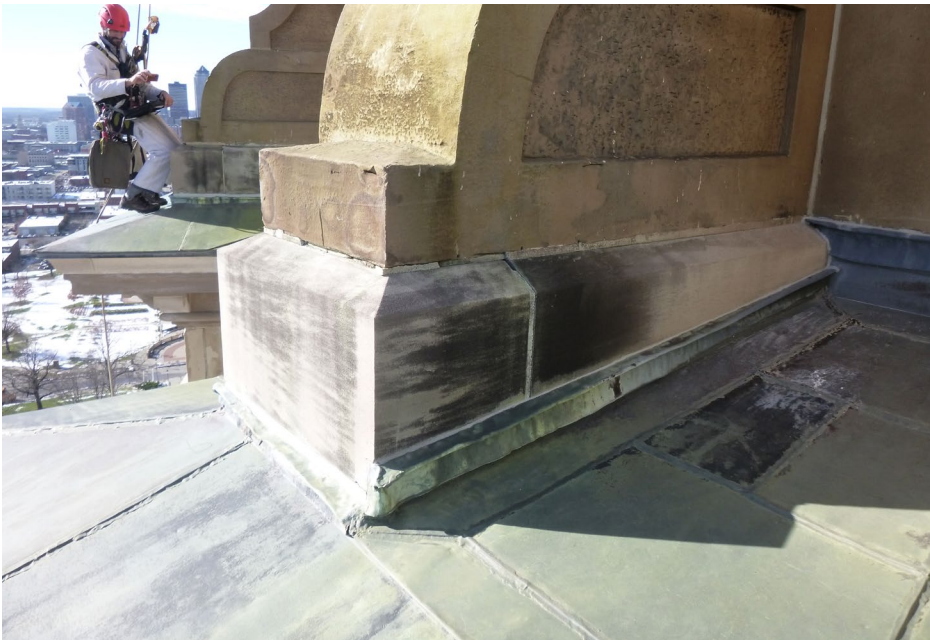
Photo 69 Stone bracket at lower cornice; note failed mortar joints at base of bracket.
