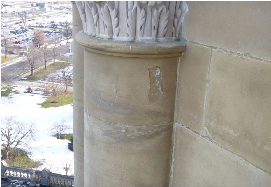
Photo 75 Typical isolated delamination.
