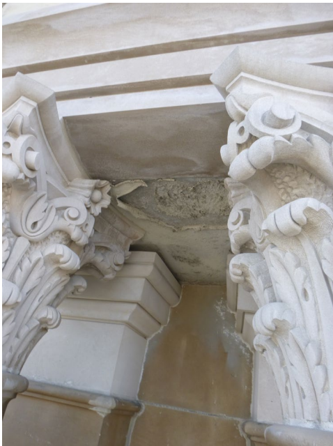
Photo 73 Exfoliation at stone soffit below lower cornice and behind pair columns.
