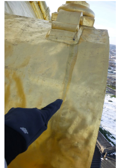
Photo 58 Water stains at hole in lead fillet at eyebrow dormer finial.
