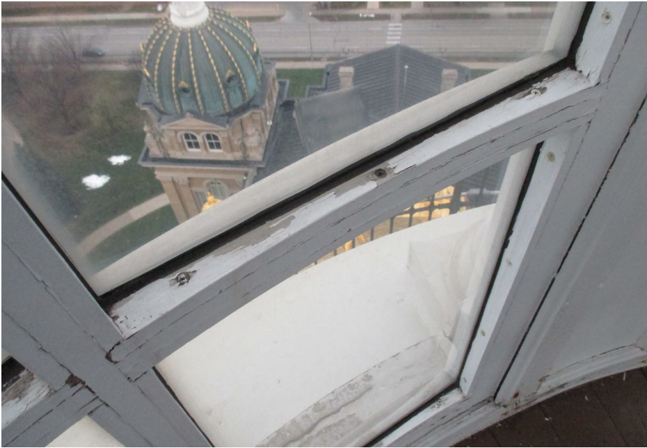
Photo 10 Deteriorated wood at lantern window midrail.
