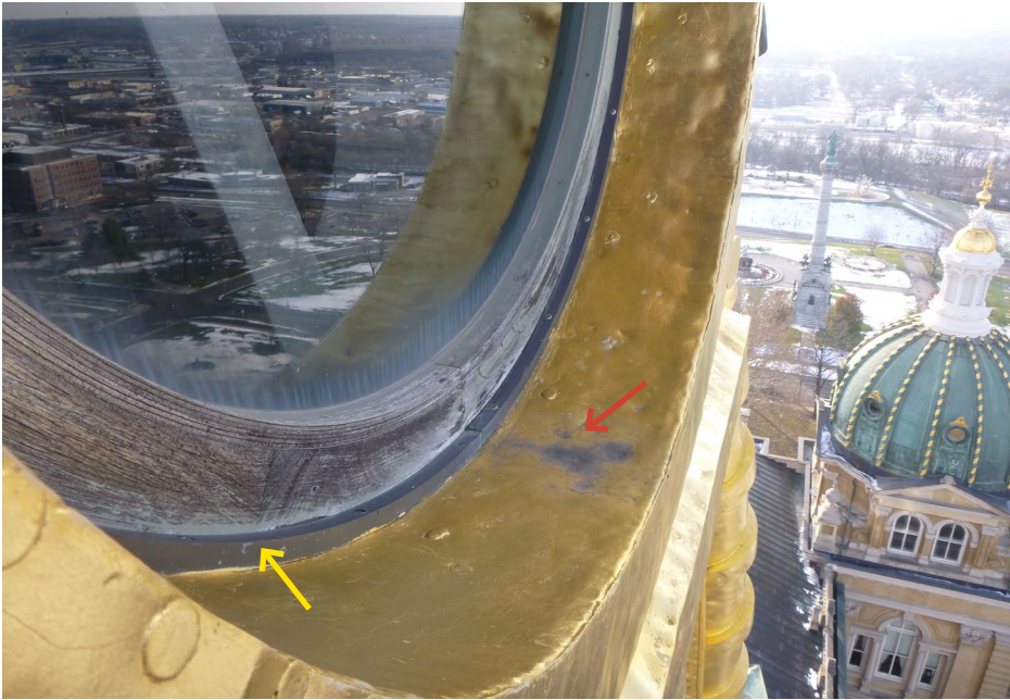
Photo 63 Wood-framed circular window with unsealed metal stop (yellow); note water stain on metal cladding in front of window sill (red).
