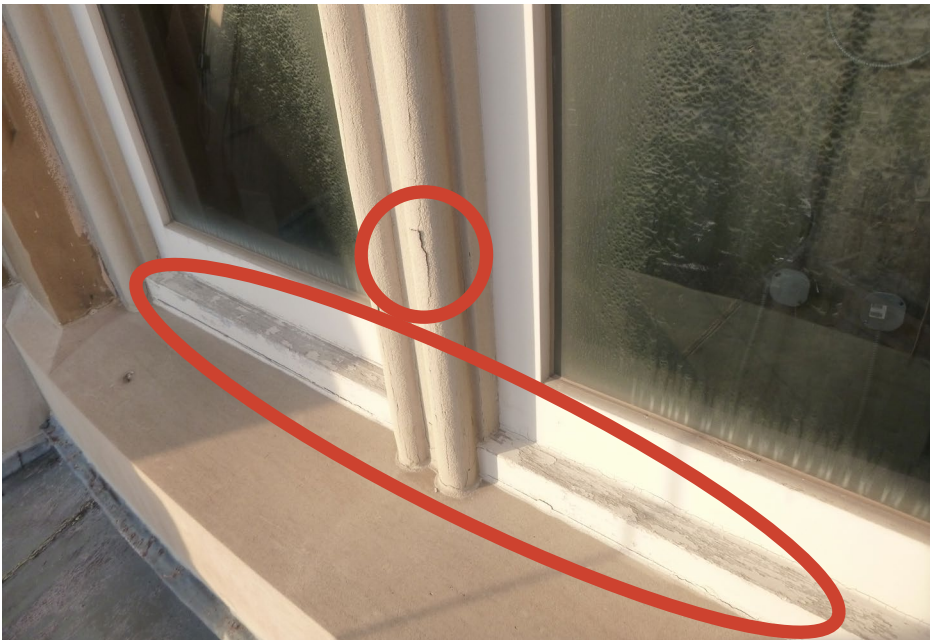
Photo 77 Typical dome window; note failing textured coating on wood mullion and sill.
