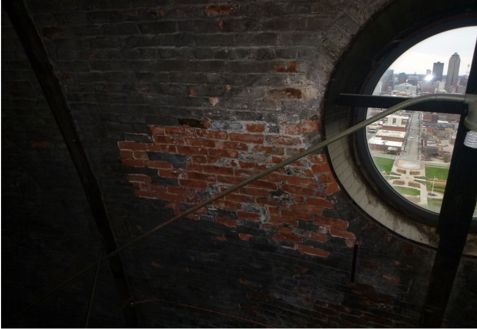
Photo 26 Brick deterioration adjacent to west window.
