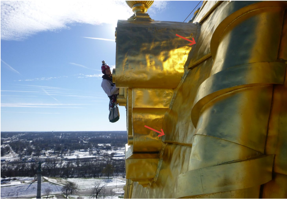
Photo 54 Typical dome eyebrow dormer viewed from the side; note continuous lead fillet along eyebrow transition to roof.
