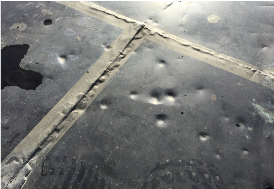
Photo 85 Stylobate level - Dented copper flatlock.
