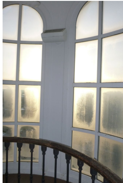
Photo 8 Lantern interior with typical condensation observed on glazing in morning.
