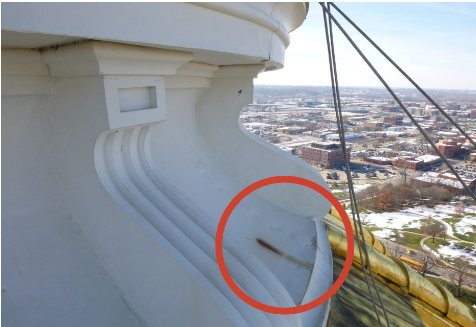
Photo 40 Rust stain on skirt cladding below a seam in soffit.
