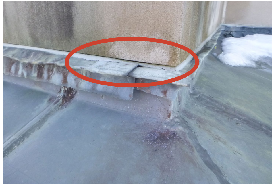
Photo 70 Failed sealant and gaps in reglet-set counter flashing at lower cornice.
