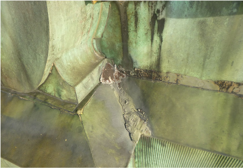
Photo 67 Typical failed solder in skyward-facing joints of copper entablature at base of dome.
