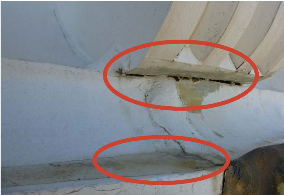
Photo 44 Typical gap at base of bracket and water on cladding below (several days after any rain/snow).
