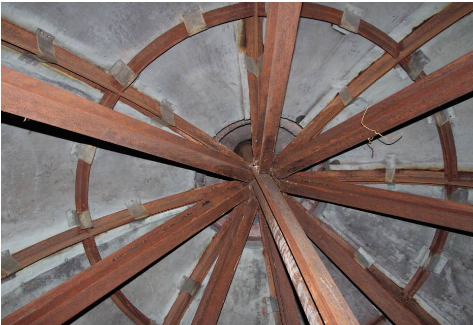
Photo 3 Metal framing and underside of lantern dome sheet metal cladding.
