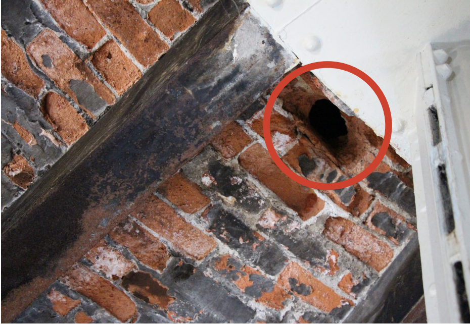
Photo 18 Spalling brick at top of dome and underside of hole noted in previous photo.
