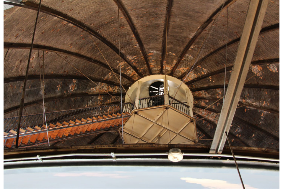
Photo 19 Stair, platform, and lantern access. Note extent of brick deterioration (red brick areas) is concentrated at top of dome.
