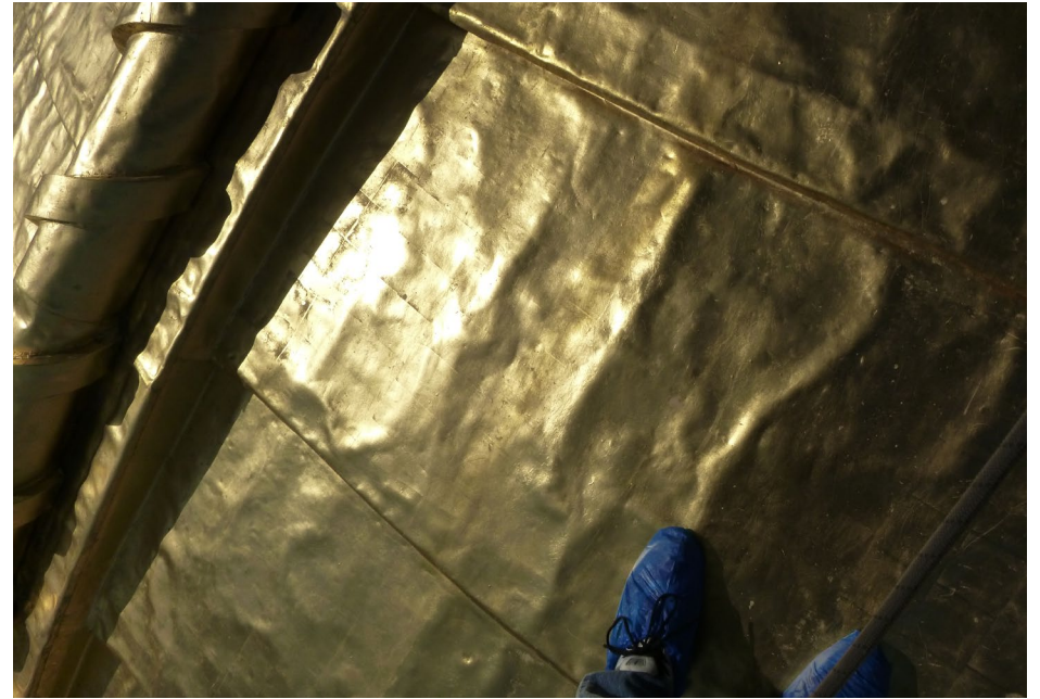
Photo 51 Buckling and waviness typically observed in dome roofing sheets.
