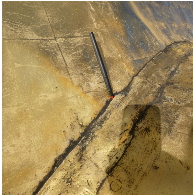
Photo 57 Separation of lead fillet at eyebrow dormer head.
