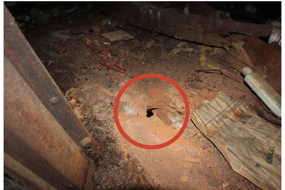
Photo 17 Top side of the dome's brick shell visible within the lantern attic; note hole in masonry.
