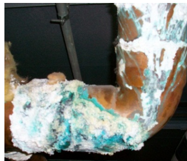
Newton Water Heater Piping
