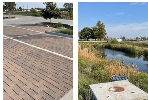
Permeable pavers and a bioretention cell in Waukeke
