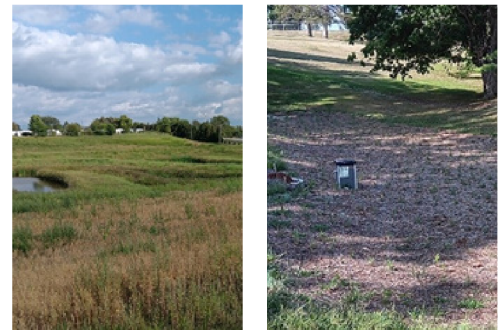
Stormwater wetland and bioretention cell in Waukon
