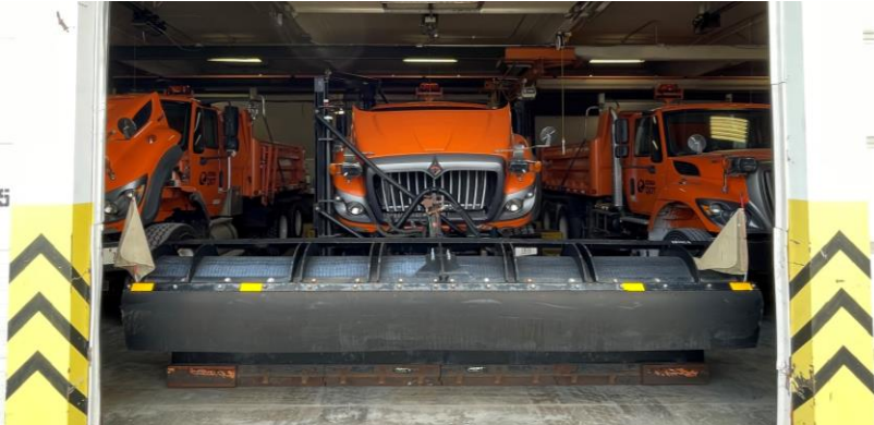
Narrow openings are difficult to enter and exit and could lead to damage to equipment and structure
