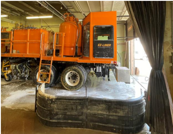
Inadequate space for vehicle size. No dedicated space for washing.
