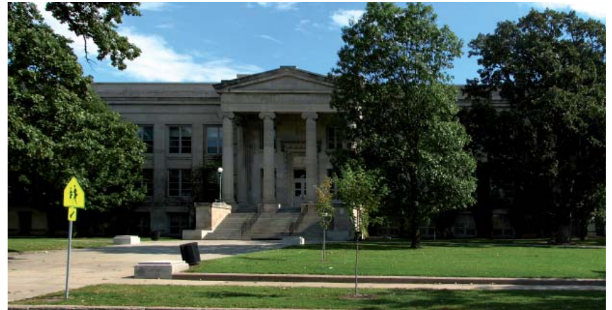
George Washington Carver Community School, top left, and East High School, above, are significant centers of community within the Capitol Park Neighborhood.
