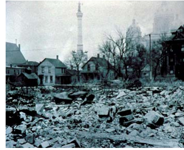
The clearing of modest structures and enhancements of the south axis greatly improved views from the trunk line trains, Left.
