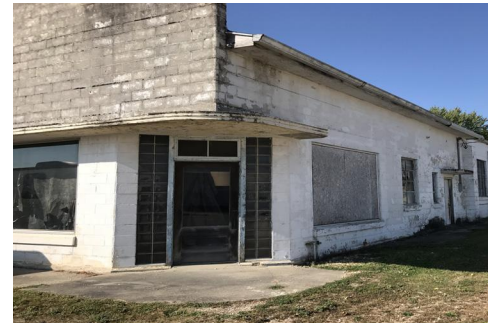
BEFORE REMODEL VACANT CAR DEALERSHIP
