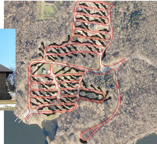
Lake Ahquabi Campground Reconstruction
