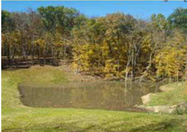
One of 29 sediment ponds installed in the park to reduce pollution to the lake.
