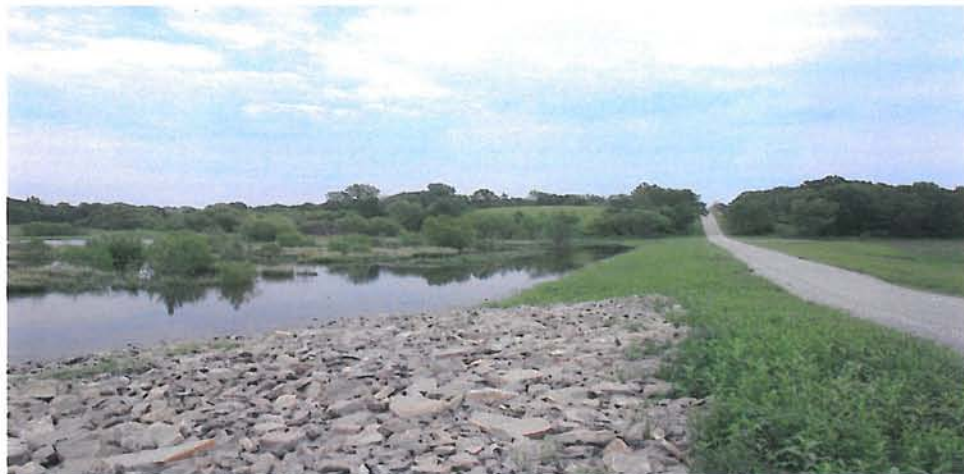
The completed Greenville Marsh Structure.
