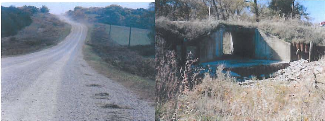
Before pictures of a 12' x 12' box culvert in bad shape in Davis County. There were several cracks, exposed re-rod, erosion problems, and safety concerns.
