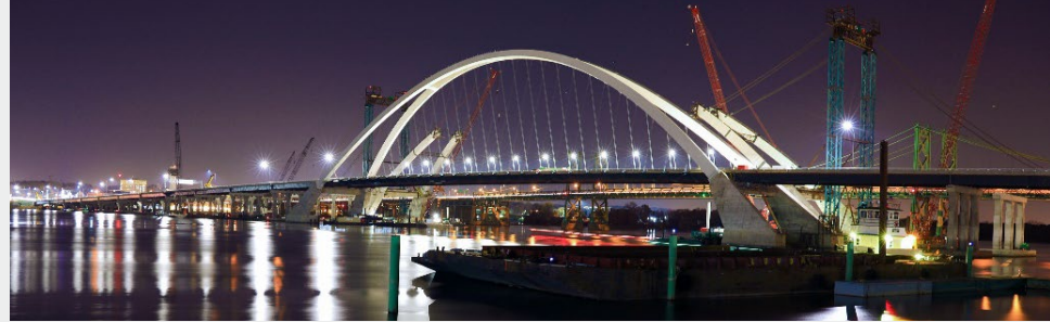
Westbound I-74 bridge construction
