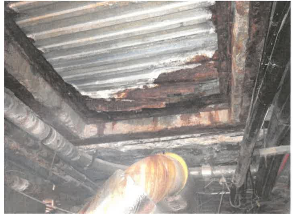
Capitol Complex Tunnels
