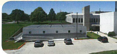
Current VDL Facility Entrance
