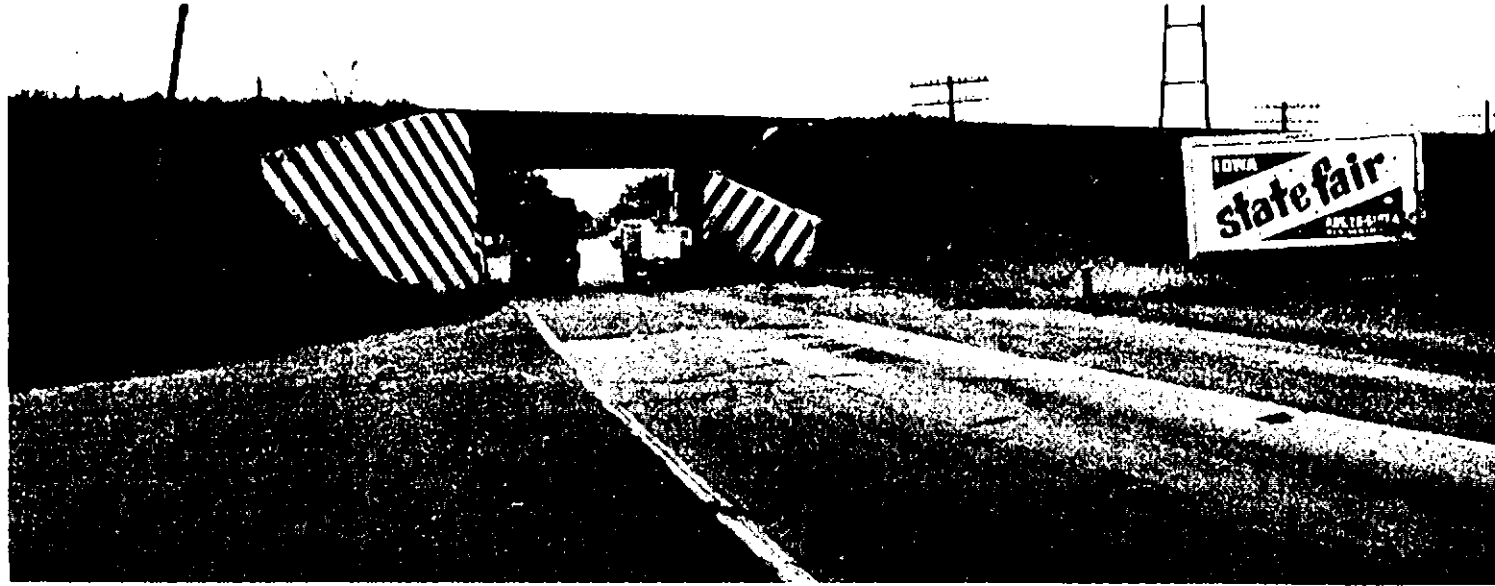
Many railroad underpasses are dangerously narrow and too frequently are approached by sharp curves.
