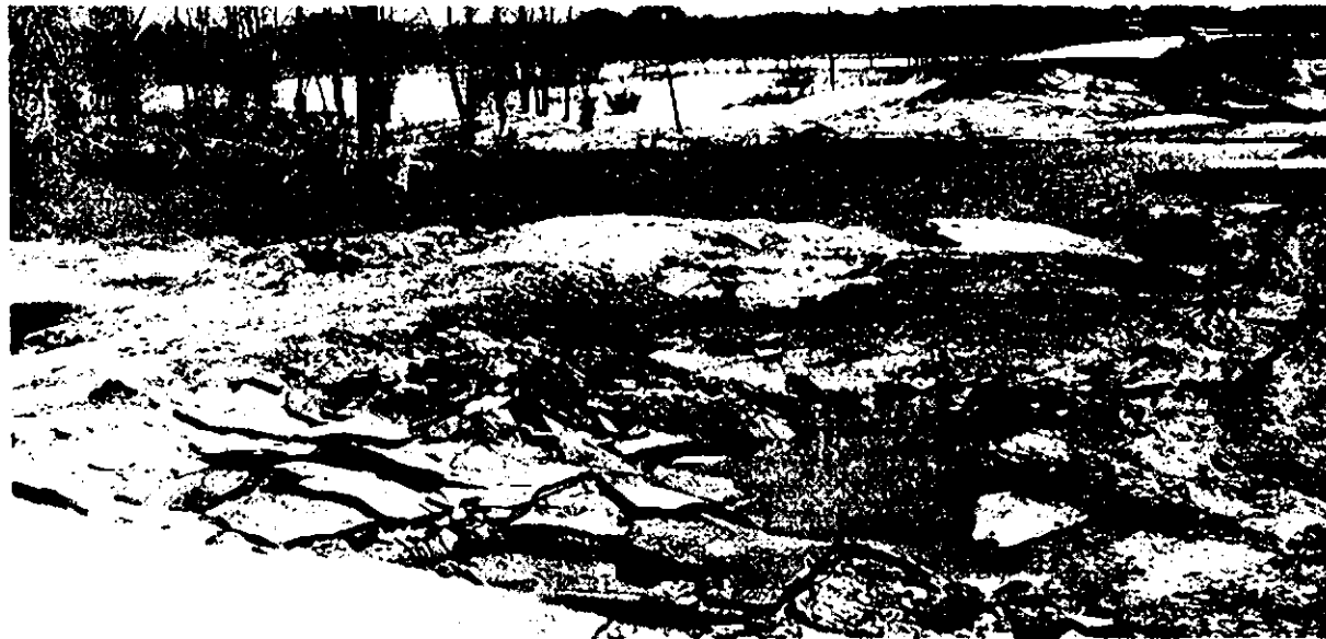
Below: The best laid plans go awry when floods, excessive freezing and thawing, or other unexpected events occur. This washout, costly to repair, shut off travel north of Vinton last April.
