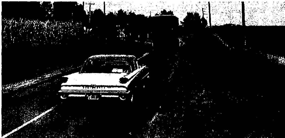
Above: One of Iowa's busiest roads is U. S. 30, yet much of it has pavement widths scarcely wide enough for trucks to pass and there are frequent no-passing zones.
