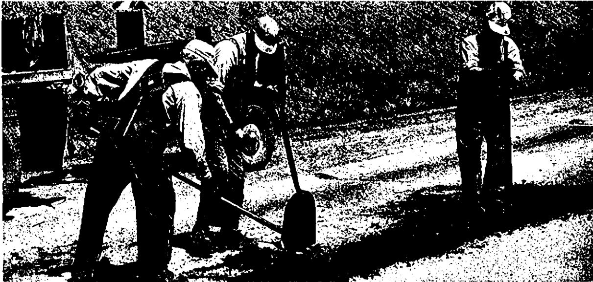
Above: The wear and tear of traffic and of weather requires constant attention—a stitch in time saves nine many times over in the case of highways.
