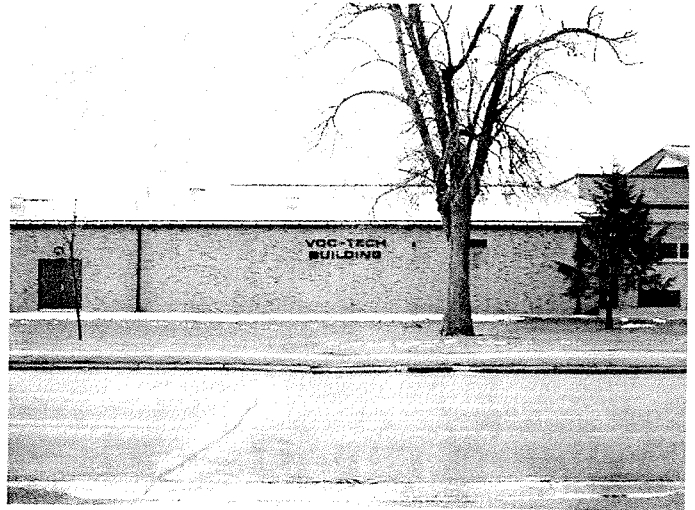
This is a frontal view of the new Voc-Tech Building built in the nineties. It is a state of the art structure containing the latest equipment.
