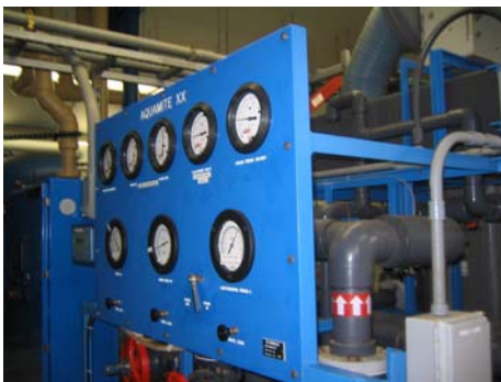
Electrodialysis reversal treatment (EDR) panel
