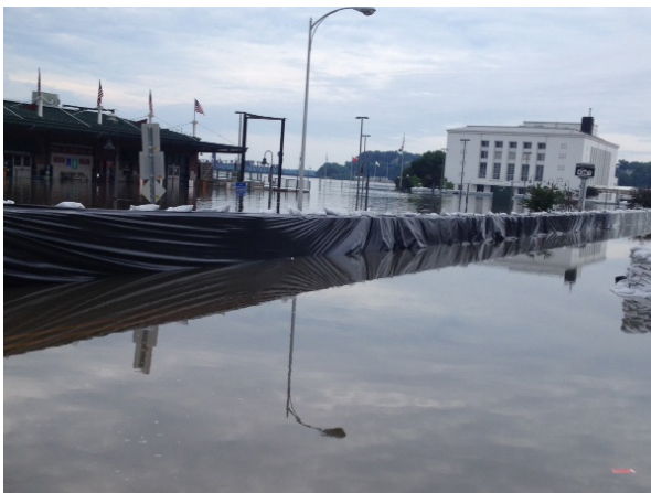
July 2014 flooding in Burlington.
