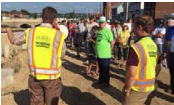
Work on the City of Dubuque's Bee Branch flood mitigation project.
