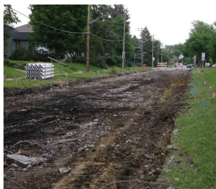
Existing non-uniform subgrade after pavement removal
