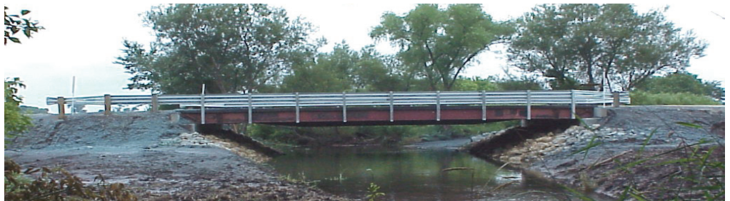
The finished Buchanan County RRFC Bridge
