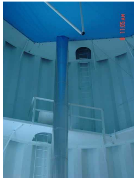
Interior of an elevated water storage tower
