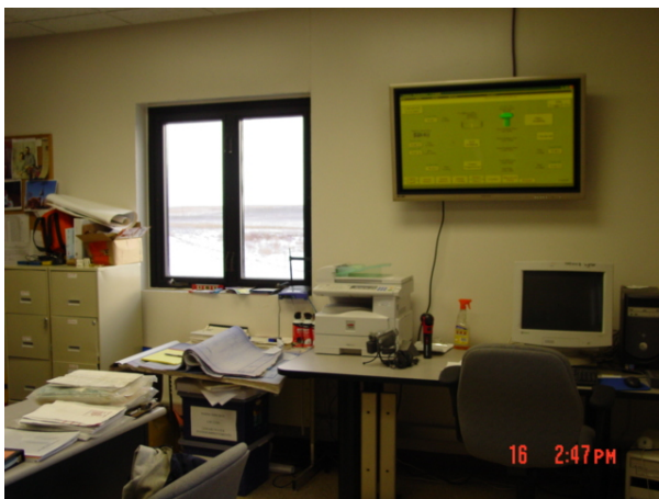
Office with computerized remote system-wide monitoring capability (typically called a SCADA system, or Supervisory Control And Data Acquisition system).
