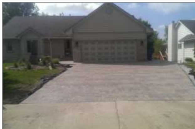
Before (left) and after (right) pictures of a permeable paver installation in the Easter Lake Watershed to reduce storm water runoff to the lake.
