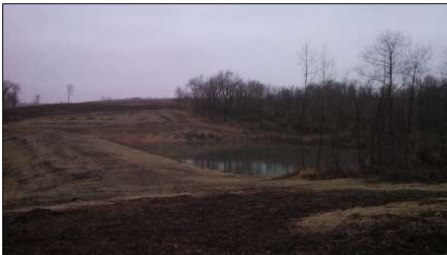
New sediment basin at Rock Creek State Park.
