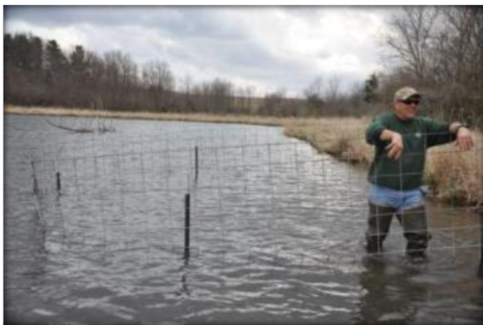
Grass carp exclusion fence is installed in Meadow Lake.
