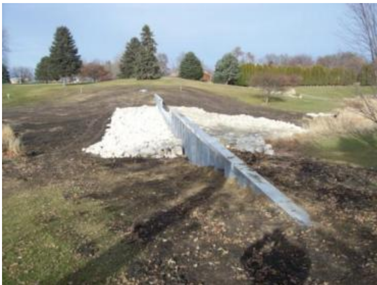
Wetland dike installed on Okoboji View Golf course.
