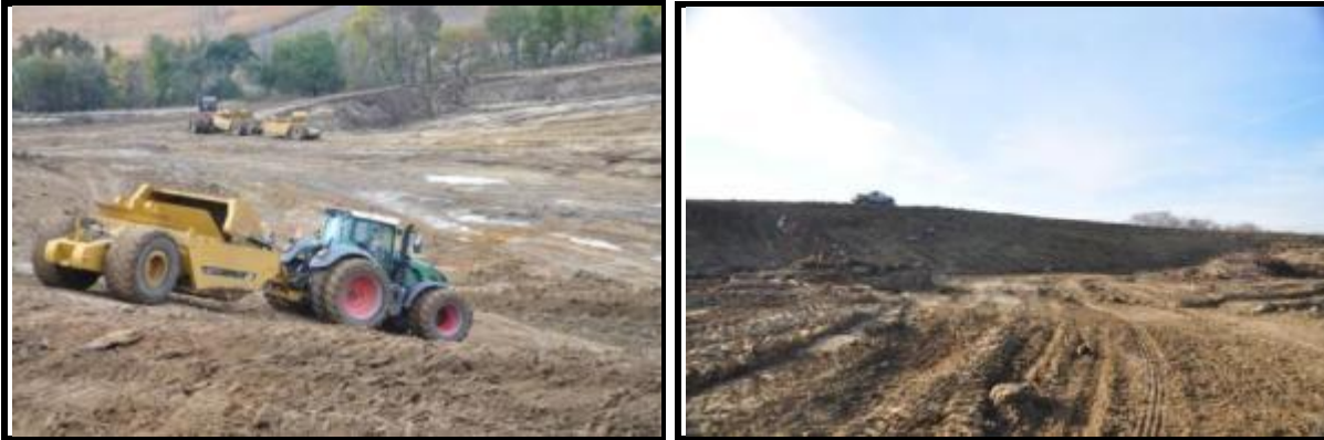
Dredge spoil containment site construction at Prairie Rose Lake, 2013.
