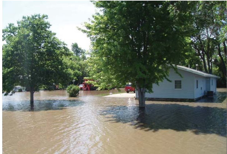
June 2014 flooding, Akron, Iowa.
