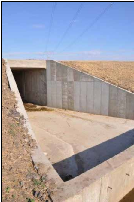
View, South Road Culvert Riser
