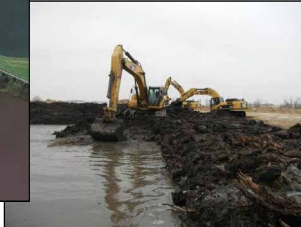
Serpentine channel excavation at the inlet of Little Storm Lake
