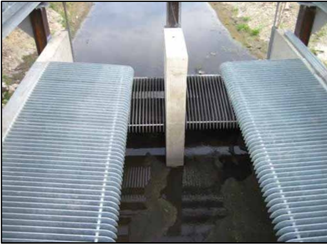
The new outlet and water control structure at Pickerel Lake (above). Fish barriers on the outlet structure at Pickerel Lake (left). These overhanging fingers allow debris to flow over the barriers but keep carp from jumping up into the lake from downstream. Note the barriers on the stop logs can move up and down with the elevation of the logs.
