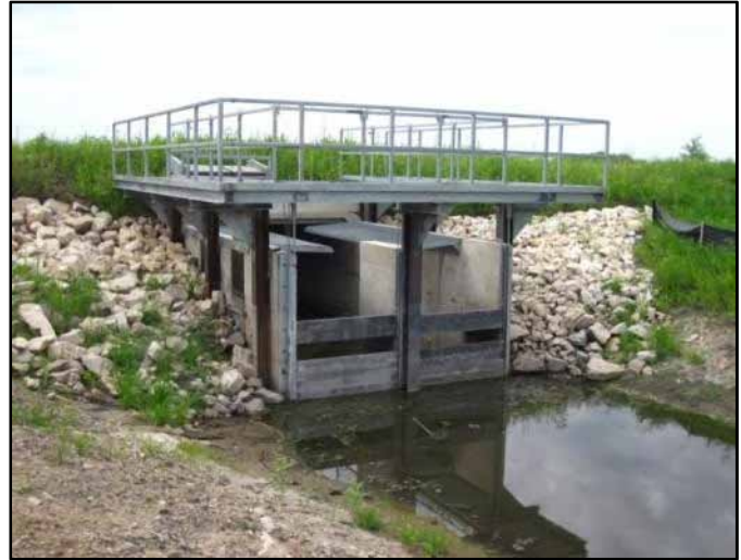
The new outlet and water control structure at Pickerel Lake (above). Fish barriers on the outlet structure at Pickerel Lake (left). These overhanging fingers allow debris to flow over the barriers but keep carp from jumping up into the lake from downstream. Note the barriers on the stop logs can move up and down with the elevation of the logs.
