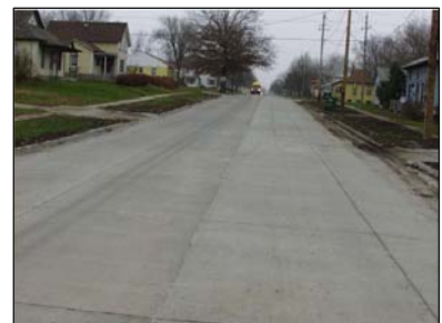
Completed Jointing Pattern
