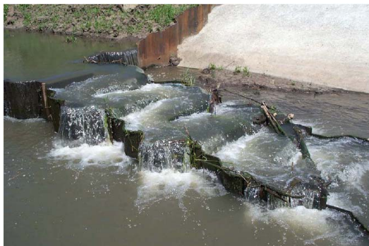
A plan/side panoramic view of a fish ladder
