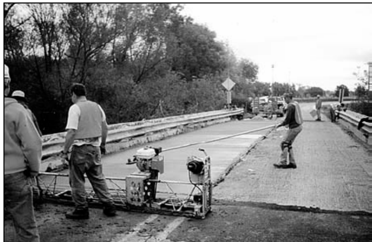
PCC Placement on the Independence Bridge
