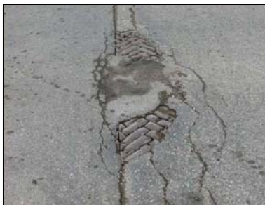
Asphalt Surface with Exposed Brick
