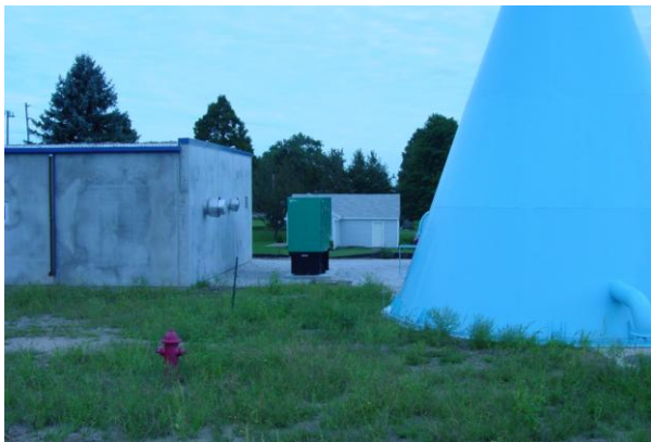
New hydrant, emergency generator, & elevated storage tower
