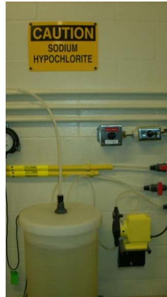
Liquid chlorine feed
