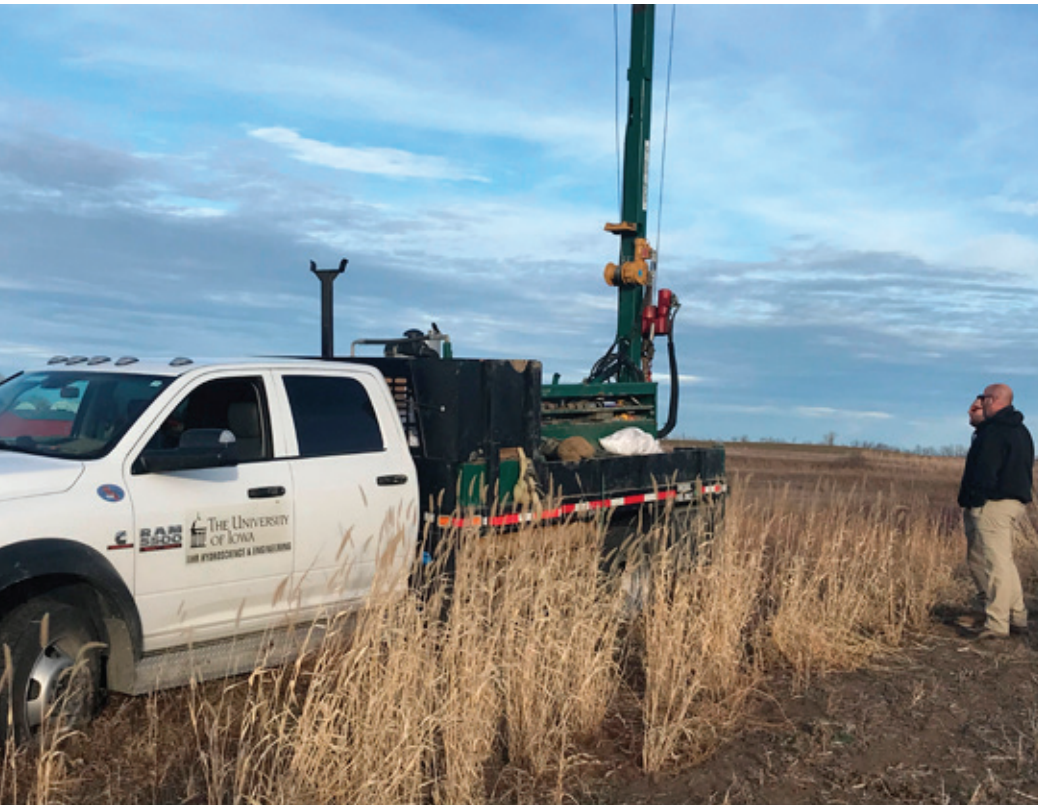
FIGURE 1 (ABOVE). Installation of a shallow monitoring well in the Iowa Great Lakes Watershed.
