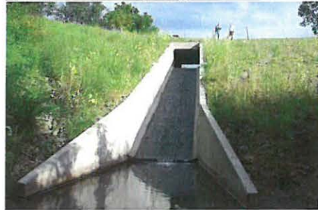
Top: 4 foot high sheet pile weir with a 1:20 gouted riprap slope in Crawford County. Bottom: RCB flume with 25 feet of fall in Fremont County.
