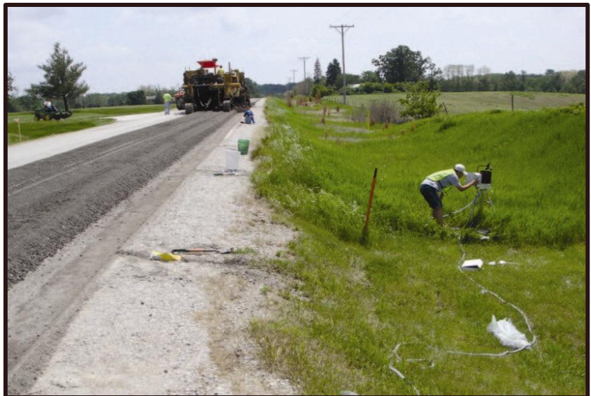
Installation of weather station
