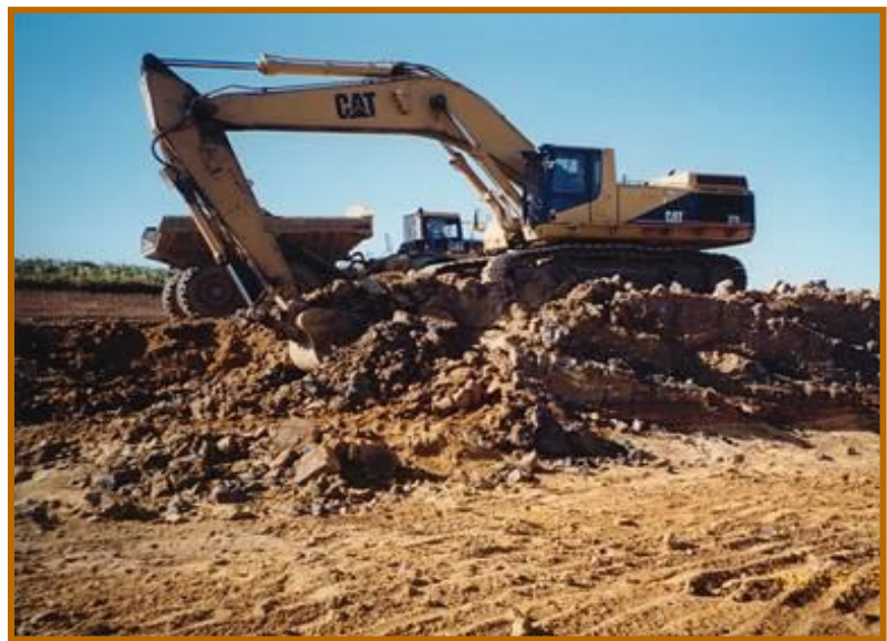
Soil mixing operation through layered soils, Des Moines, Iowa Photo: Vern Schaefer, Iowa State University/CCEE
