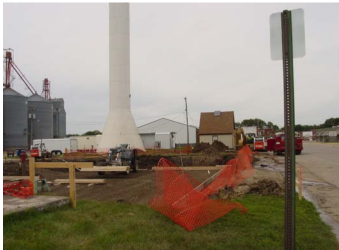
Beginning Construction of a new Reverse Osmosis Treatment Plant
