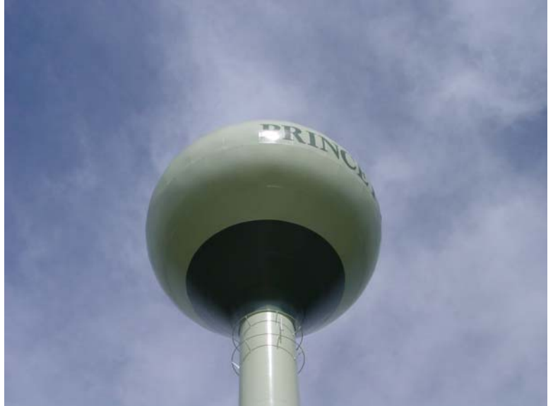
New Elevated Storage Reservoir
