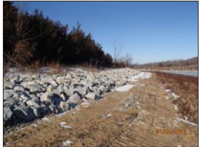
Shoreline stabilization of regions with significant erosion
