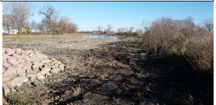
Completed construction on Nebowa Bay in Fall 2016
