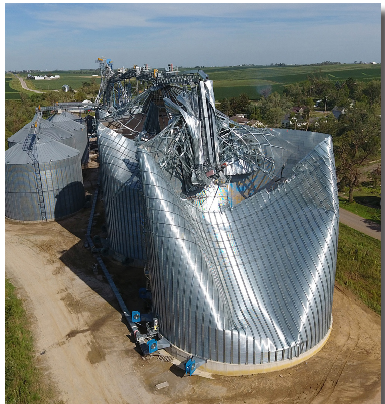
Tama County grain bins collapsed in the derecho storm. Photo: Kip Ladage, Bremer County Emergency Management
