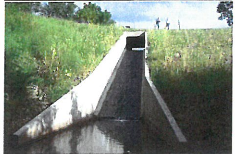
Top: 4 foot high sheet pile weir with a 1:20 grouted riprap slope in Crawford County. Bottom: RCB flume with 25 feet of fall in Fremont County.
