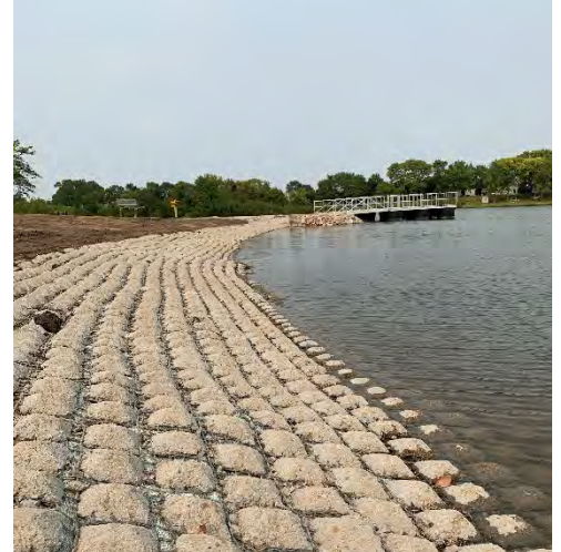
Flexamat (pictured here) was installed along the shoreline in 2020 to protect the lake from erosion and provide access to the water.
