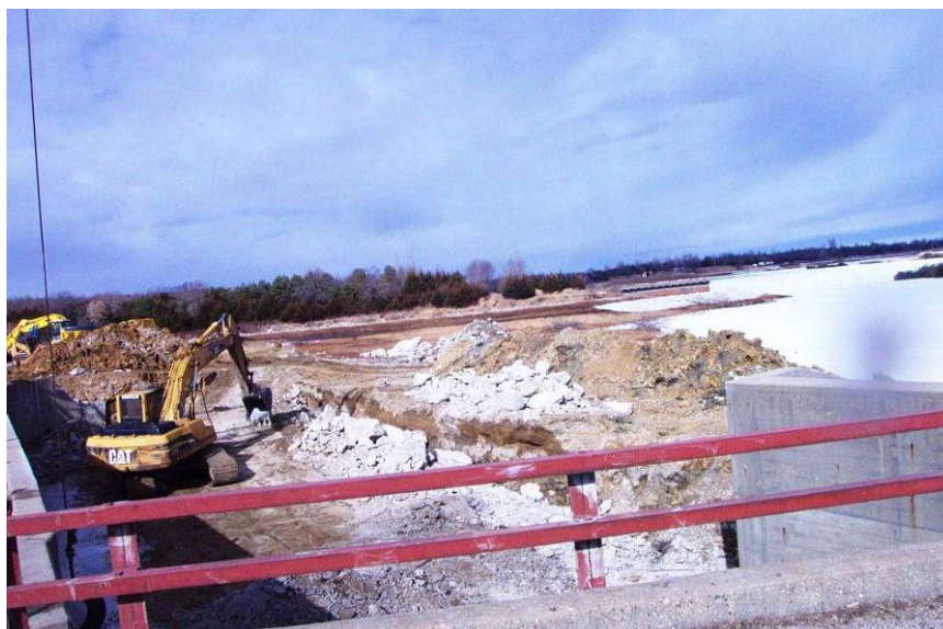
Green Valley Lake (Union Co.) spillway repair and modification project
