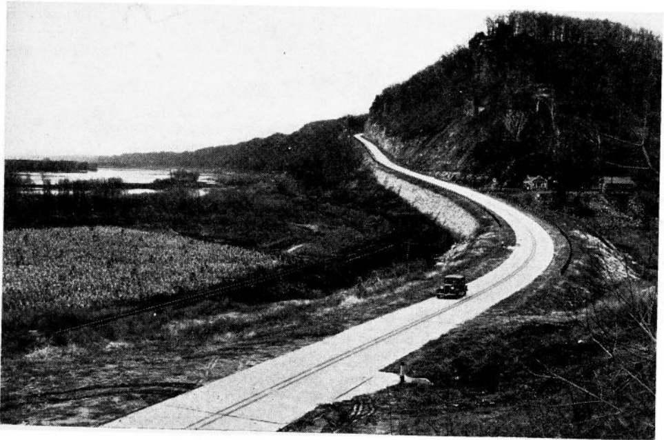
Federal Highway 52 Near Guttenberg
