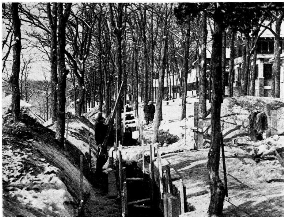
Great Lakes WPA Sewer Project
