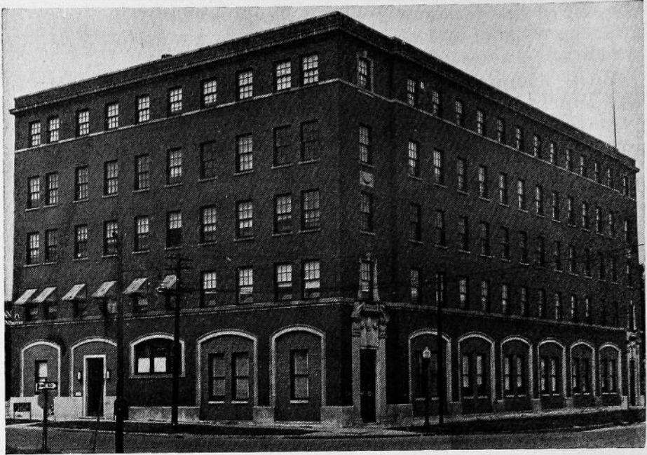
OFFICE AND LABORATORY BUILDING
