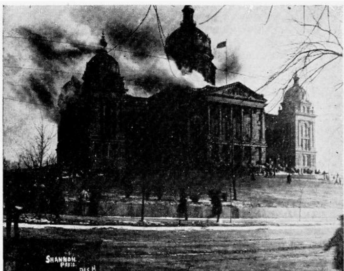
State Capitol on Fire January 4, 1904, the north wing of the Capitol was badly damaged by fire of unknown origin.
