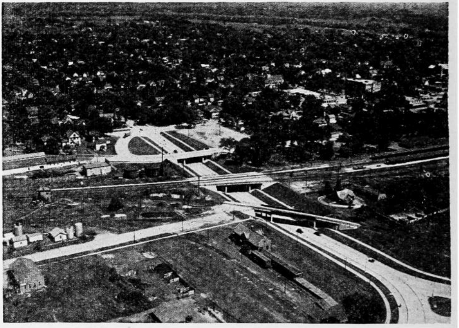
Subway and Traffic Separation Project at Ames
