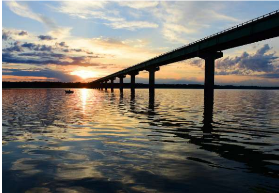
High Trestle Trail Bridge
