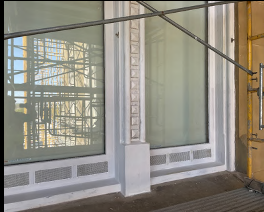
AFTER PAINT AND SAND FINISH
