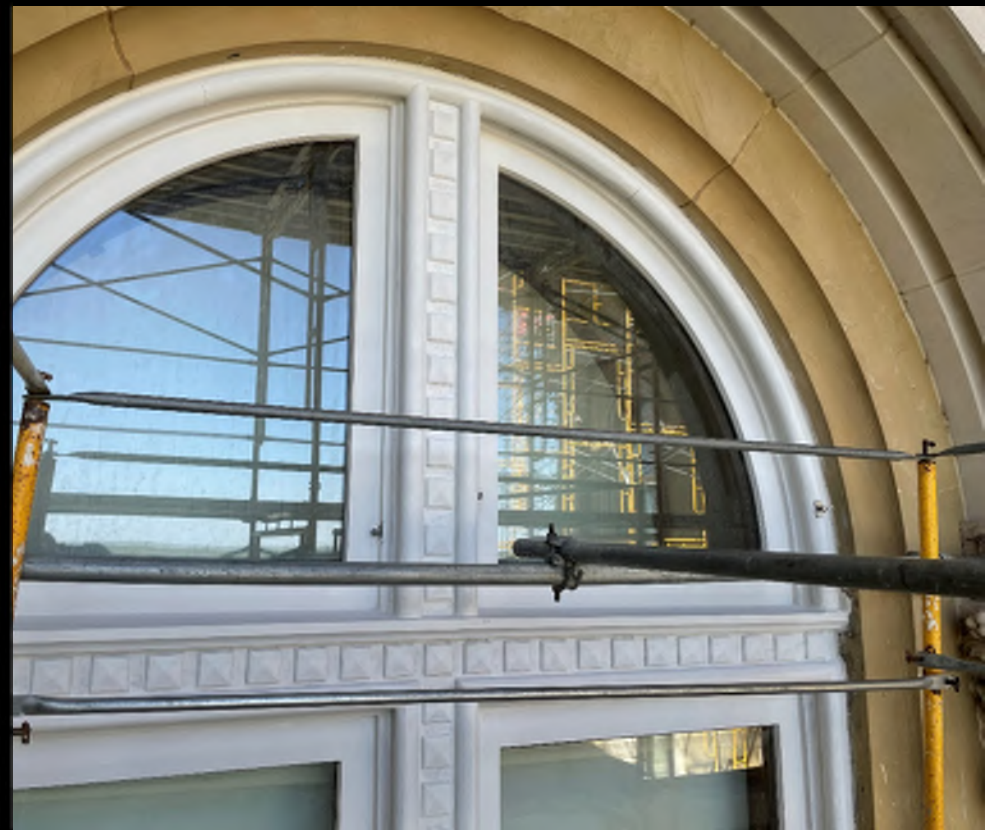
AFTER PAINT AND SAND FINISH
