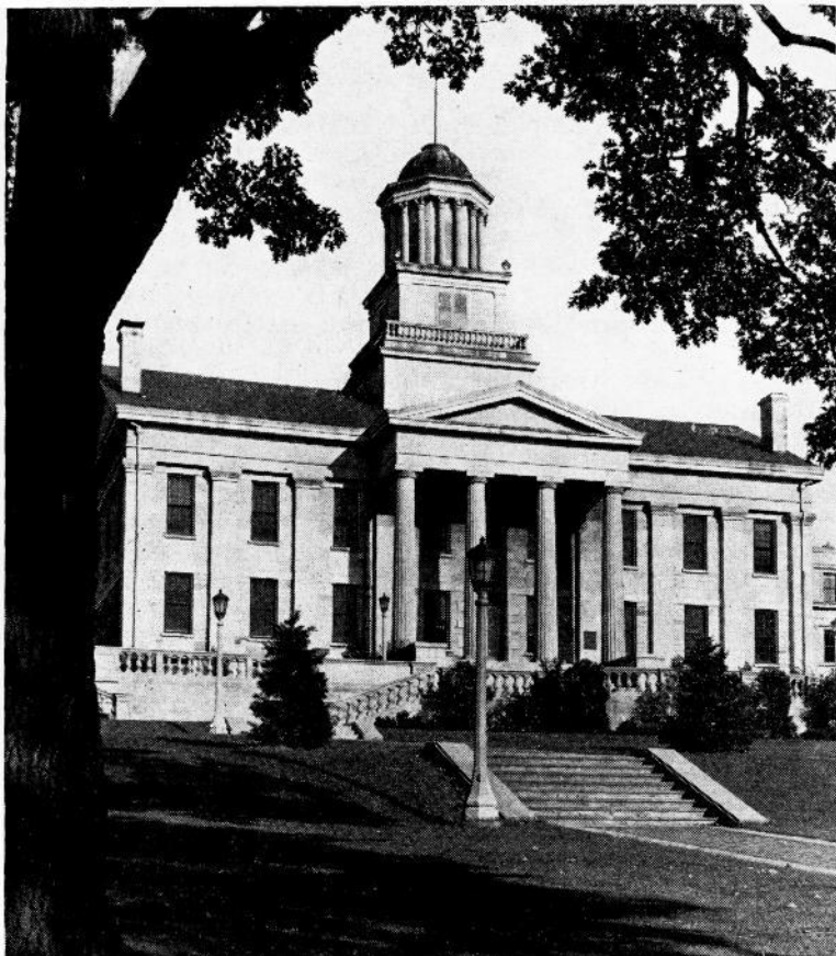
Former State Capitol Building
