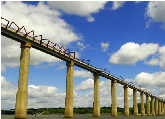
High Trestle Trail Bridge
